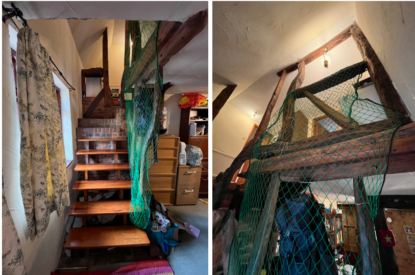
Fig. 19 - Photos of the existing stairs.
