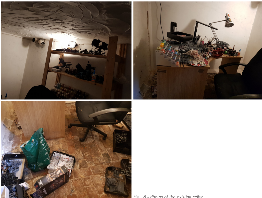
Fig. 18 - Photos of the existing cellar.
