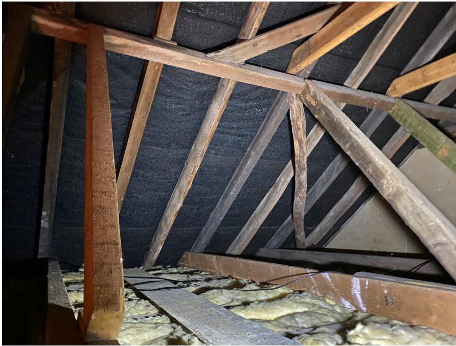
Fig. 13 - Photo of the loft space above the proposed bedroom 1.
