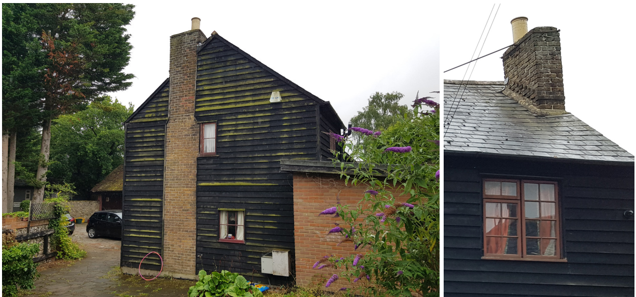
Fig. 12 - Photos of Chimney B.
