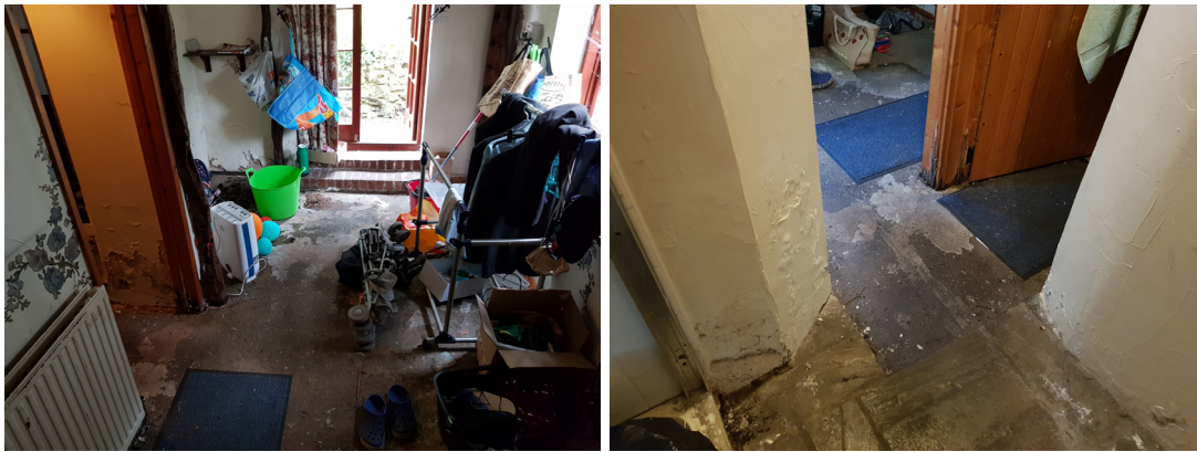
Fig. 17 - Photos of the existing cellar.
