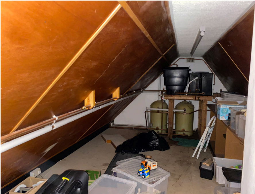
Fig. 16 - Photo of the loft space under the main clay tile roof.
