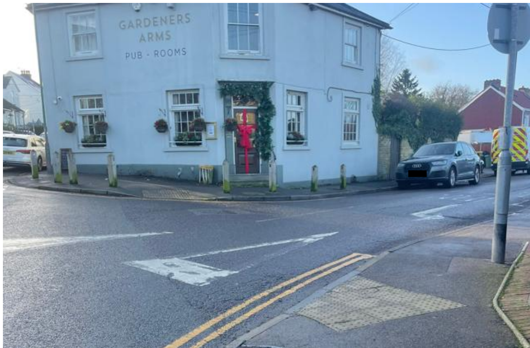
FIGURE 2-20: SCHOOL LANE CROSSING TO FORGE LANE (COURTESY OF DHA)
