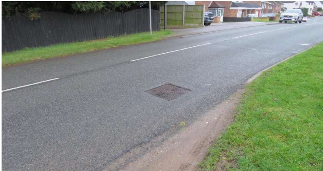
Photo 1: Cover has sunk 15-20mm
