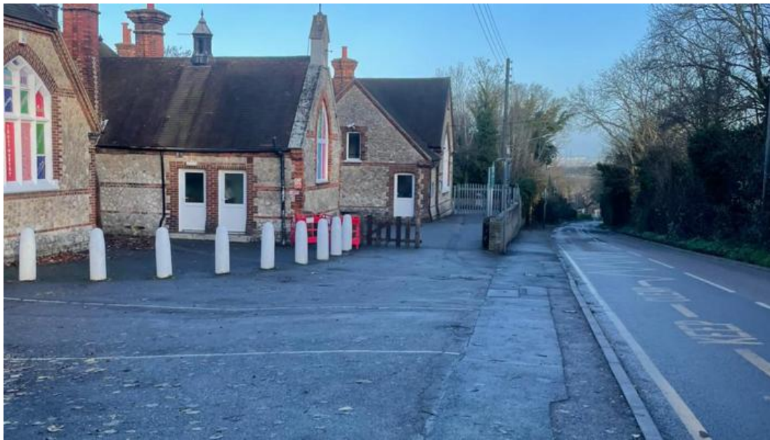
FIGURE 2-3: SCHOOL LANE ADJACENT TO PRIMARY SCHOOL (COURTESY OF DHA)
