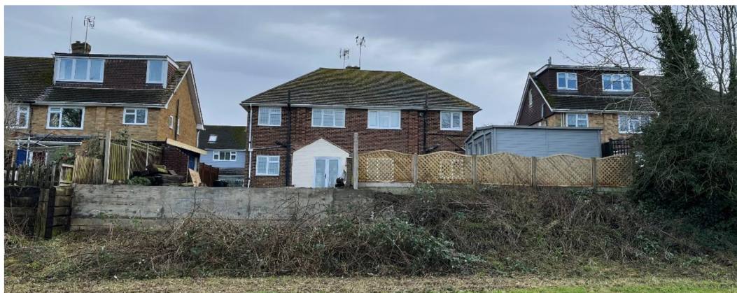
Rear of No.40
