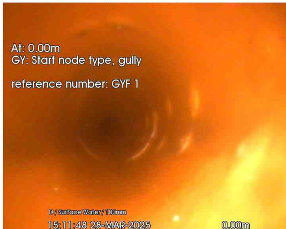
GYF 1_0-00m_151148.jpg, 00:00:02, 0.00 m Start node, gully, reference: GYF 1
