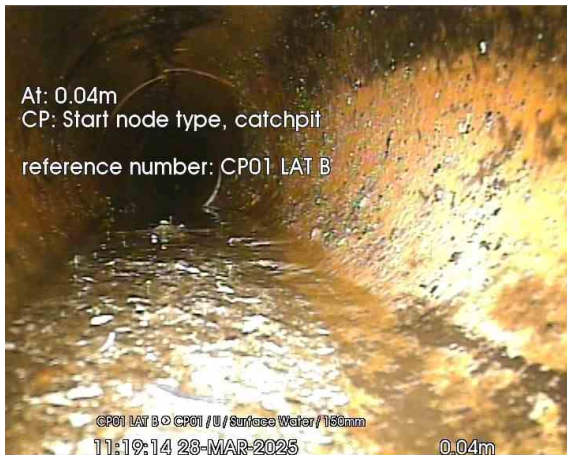
CP01 LAT B_0-04m_111914.jpg, 00:00:00, 0.04 m Start node, catchpit, reference: CP01 LAT B
