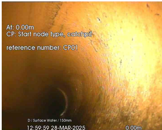
CP01 DS_0-00m_125959.jpg, 00:00:00, 0.00 m Start node, catchpit, reference: CP01
