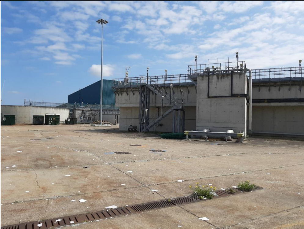
5. Effluent Treatment Plant Looking E.
