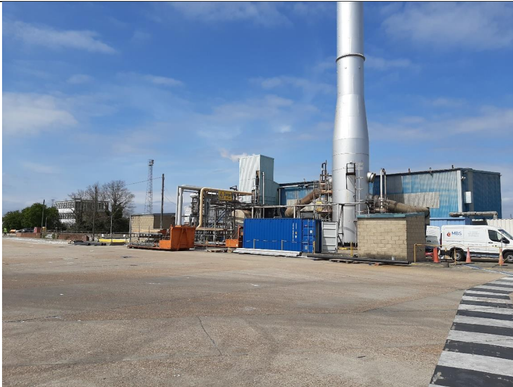
1. Boiler House Looking NW.
