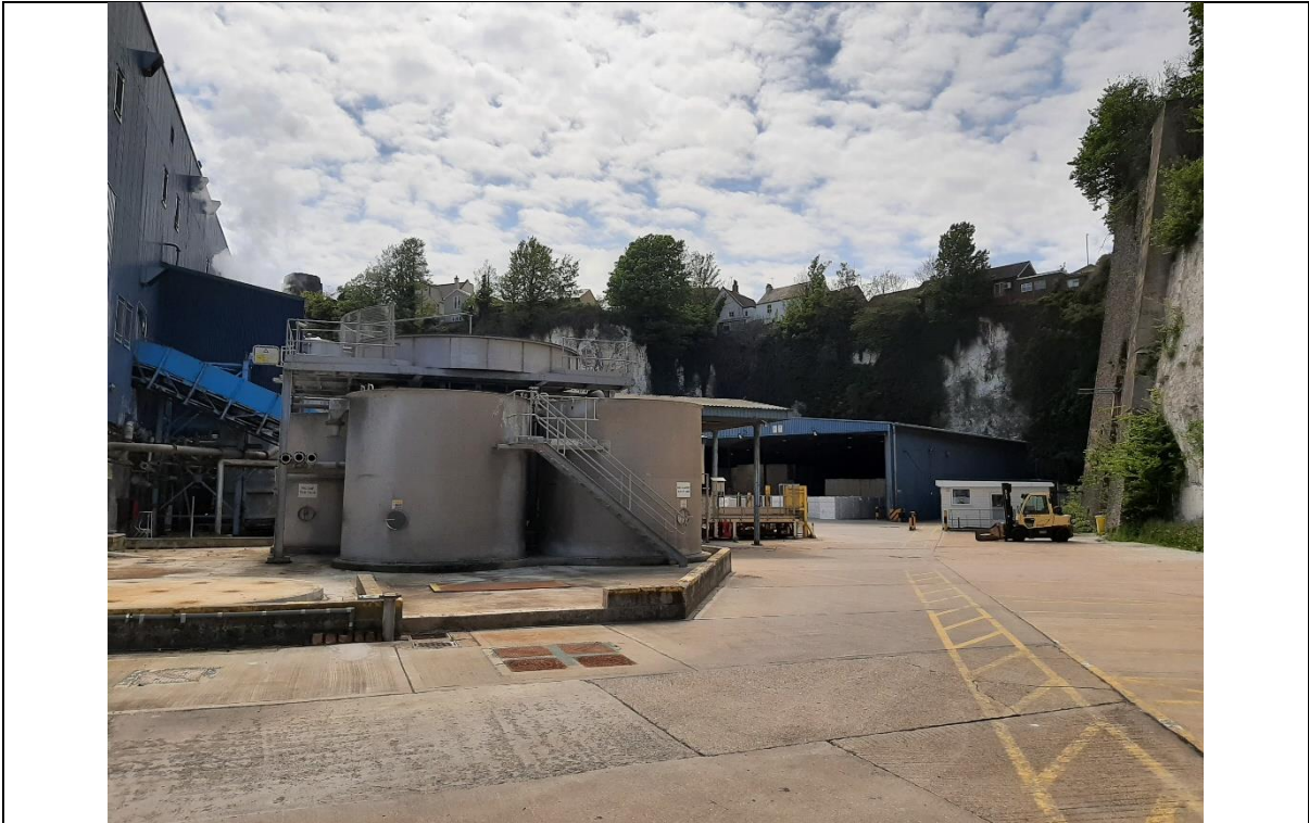
7. Storage tanks in southern area looking SE.
