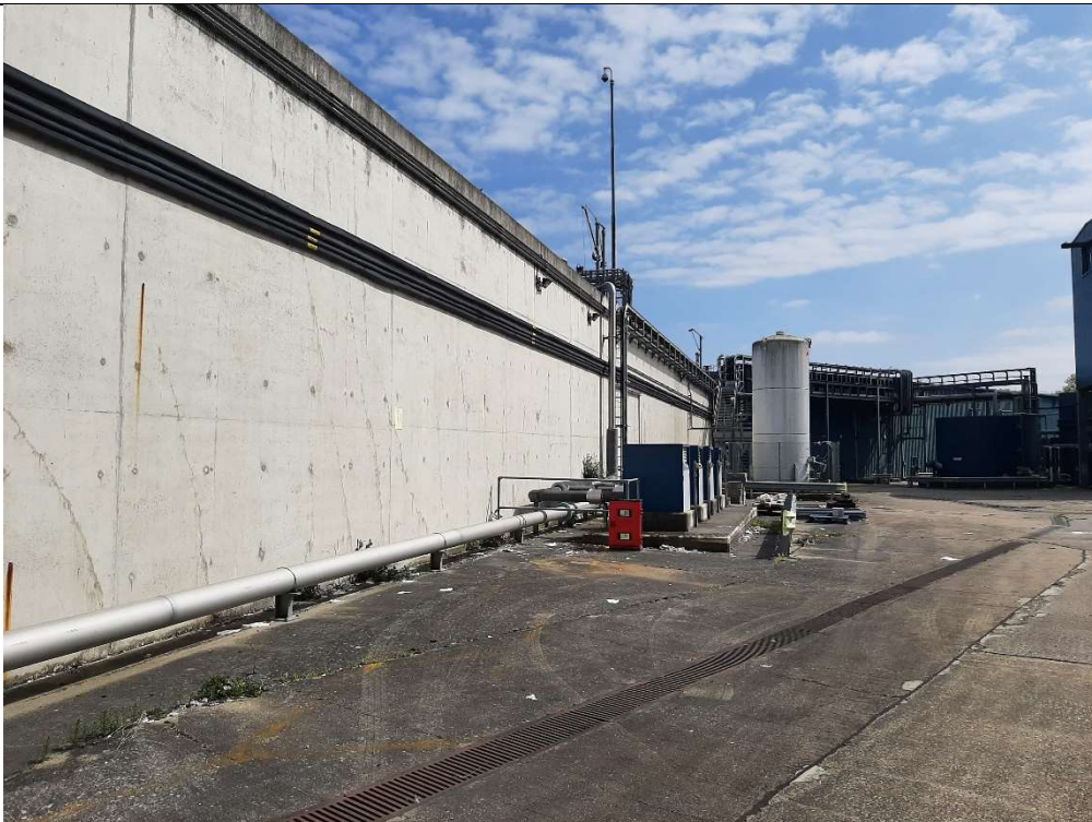
6. Effluent Treatment Plant Looking SE.
