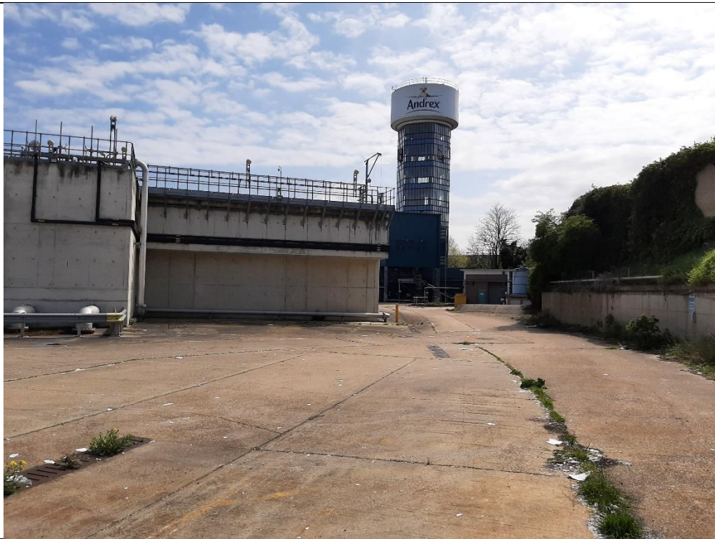
4. Effluent Treatment Plant and Water Tower.
