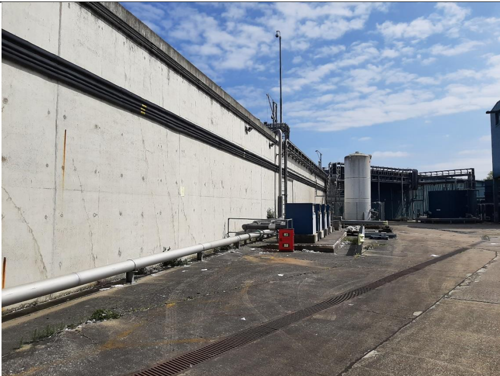
6. Effluent Treatment Plant Looking SE.
