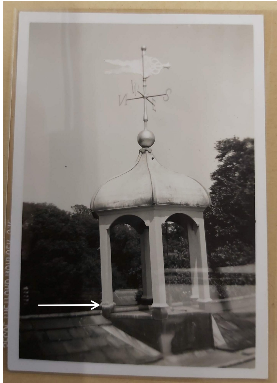
Historic photograph showing timber flashing covers
