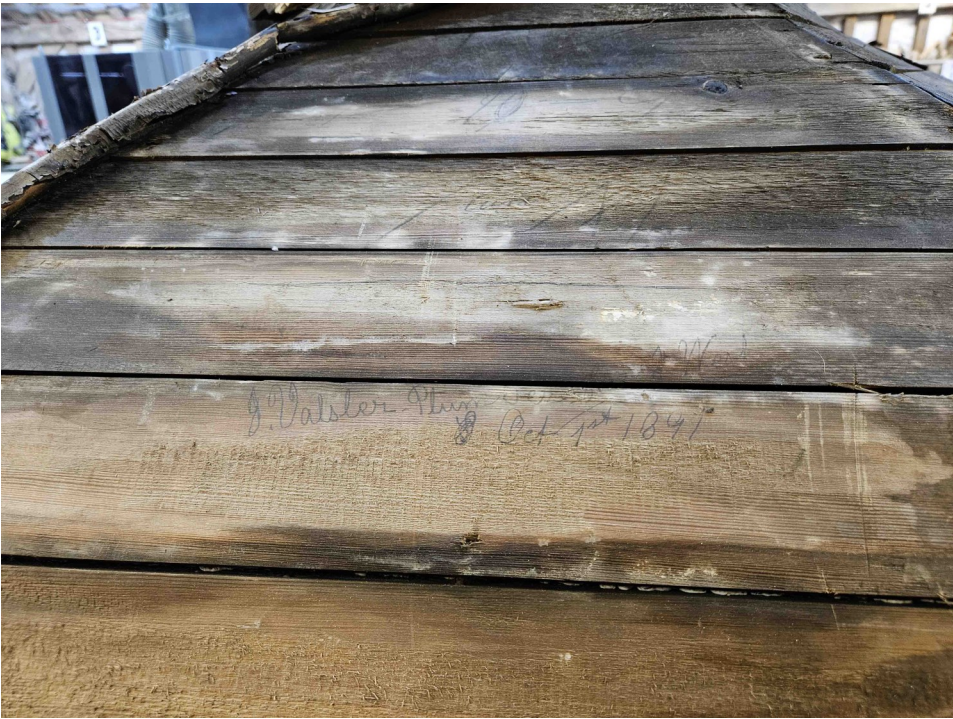
Roofing boards with inscription: J Vasler plumbers: Oct 1st 1897
