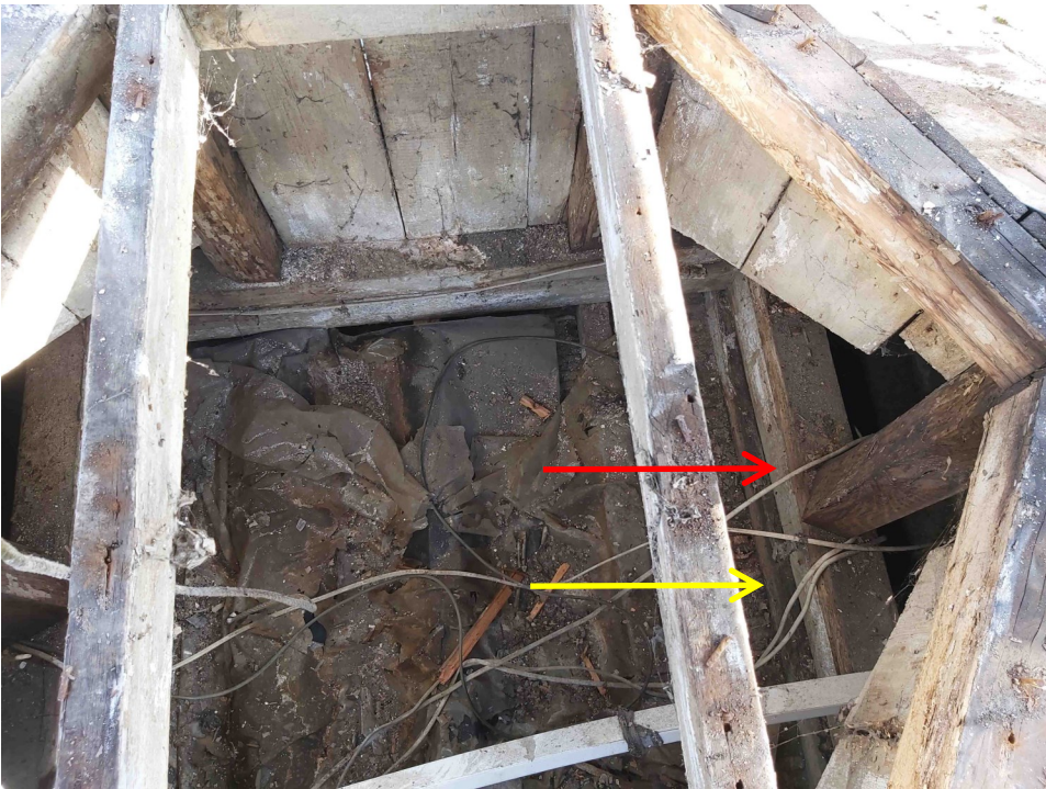
Red arrow: 'Newer' base frame (after 1860) resting on top of Yellow arrow: original base frame
