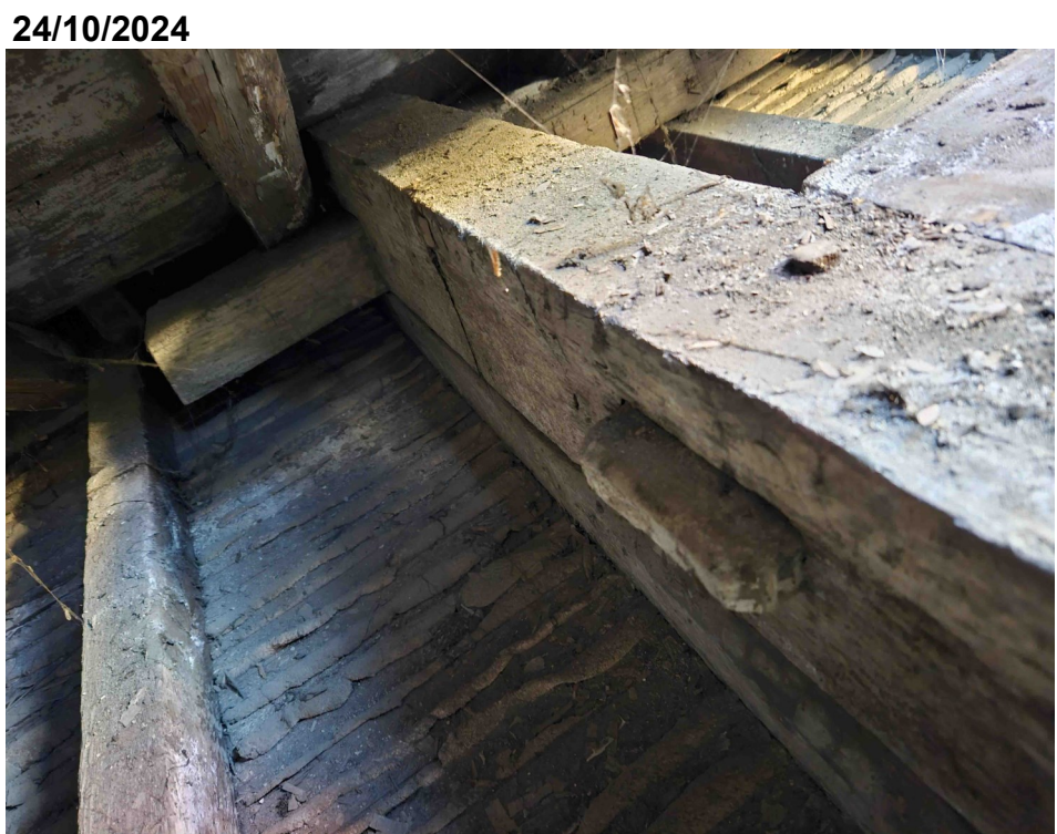
Original base frame resting on ceiling joists
