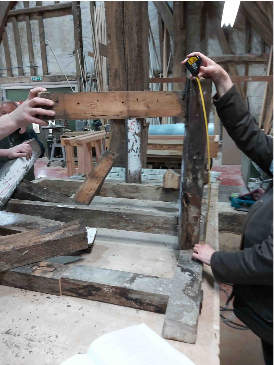
Sorting through cut frame and post connections
