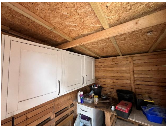
Photograph 5. Interior of B2
