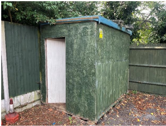
Photograph 1. Exterior of B1
