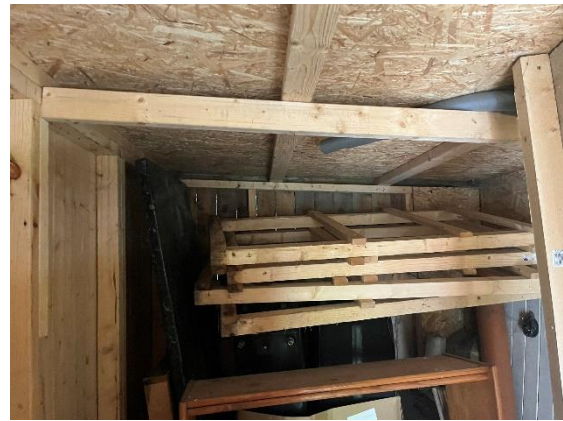
Photograph 2. Interior of B1
