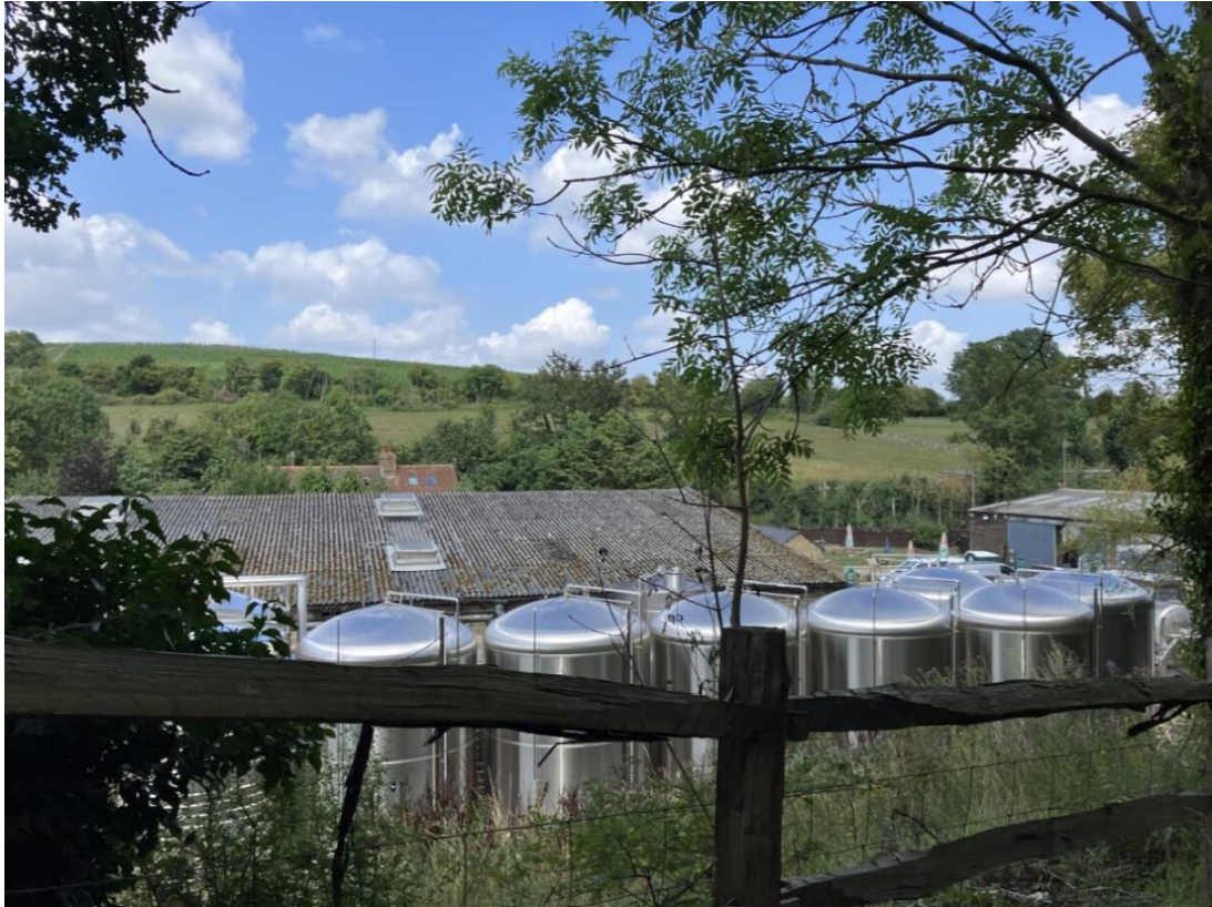
FIGURE 2-2: VIEW OF THE SITE AS EXISTING FROM CUTTERS RIDGE ROAD
