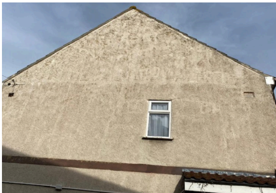
West elevation gable detail
