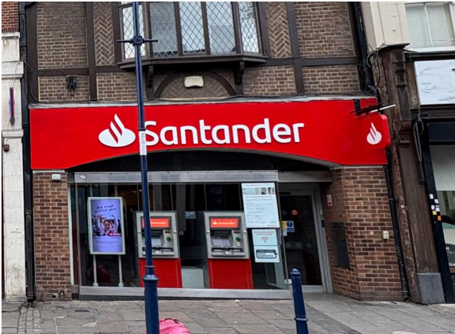
Image 6 Nearby Shop Front with raised letters , LED light & Projected Side sign
