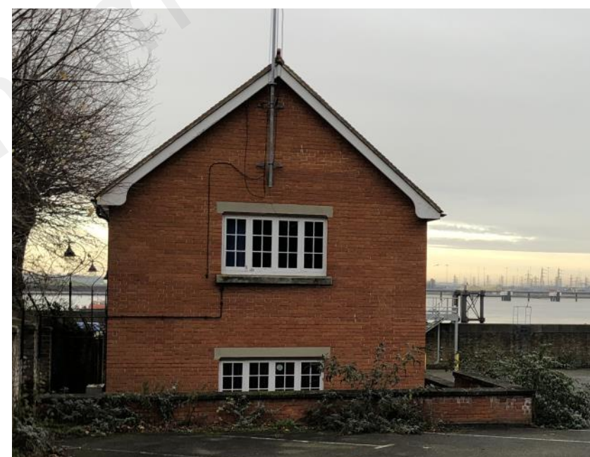
The rear Boathouse elevation.
