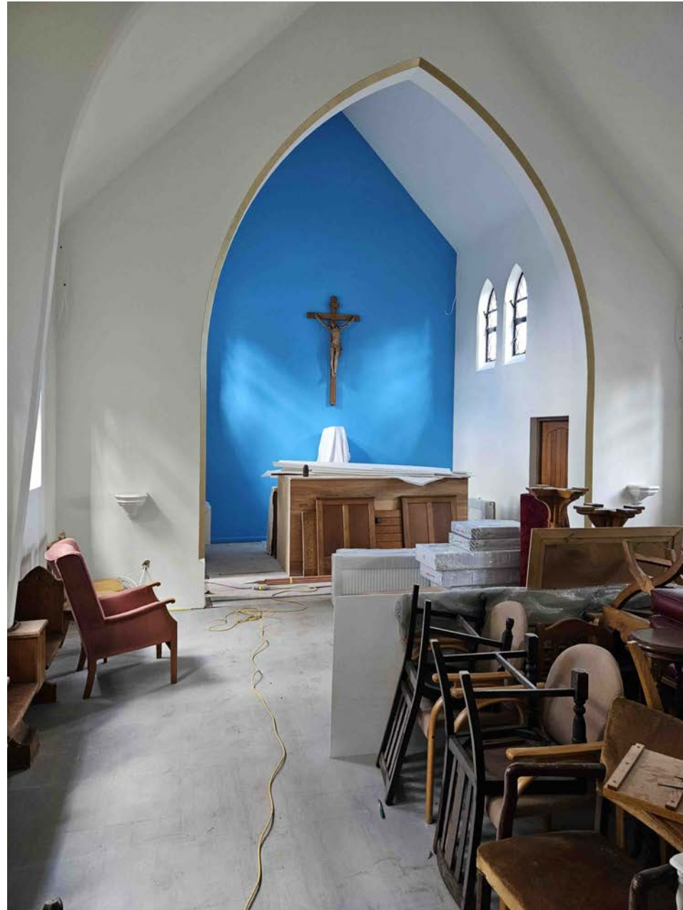
St Joseph's Chapel at the convent undergoing refurbishment
