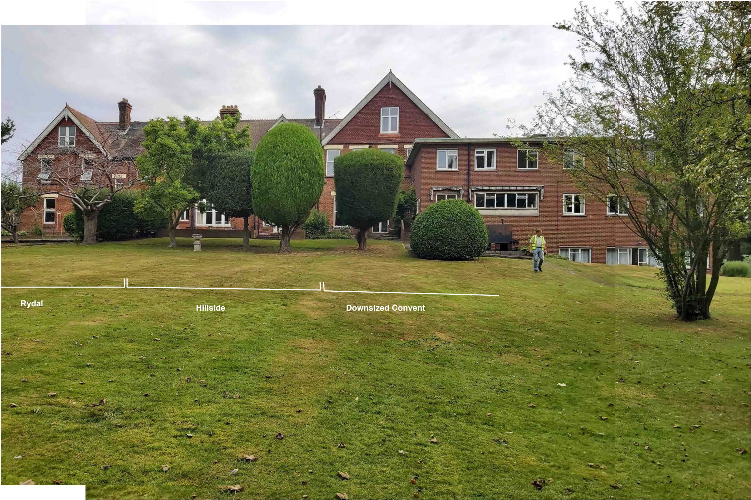
Rear elevation before refurbishment works began on the downsized Convent
