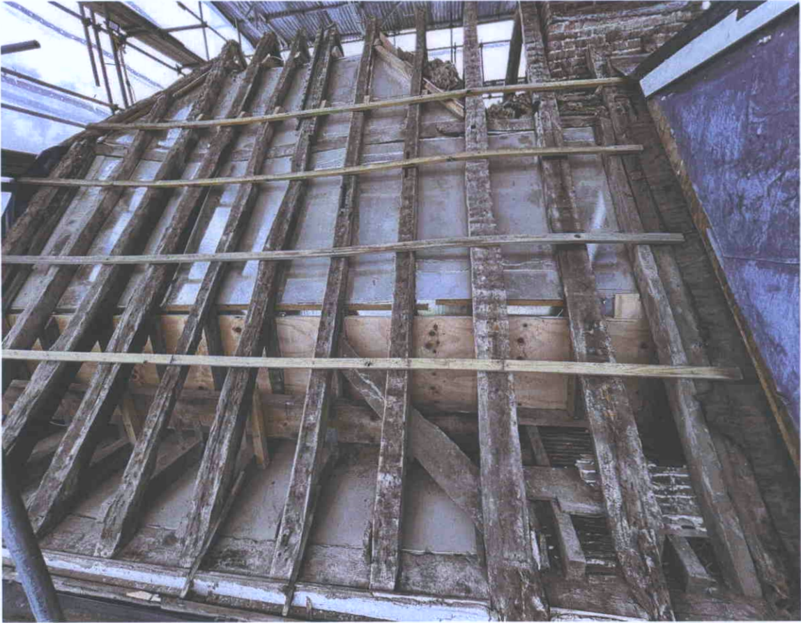
Bay 1, bay 2 at chimney and dormer south
