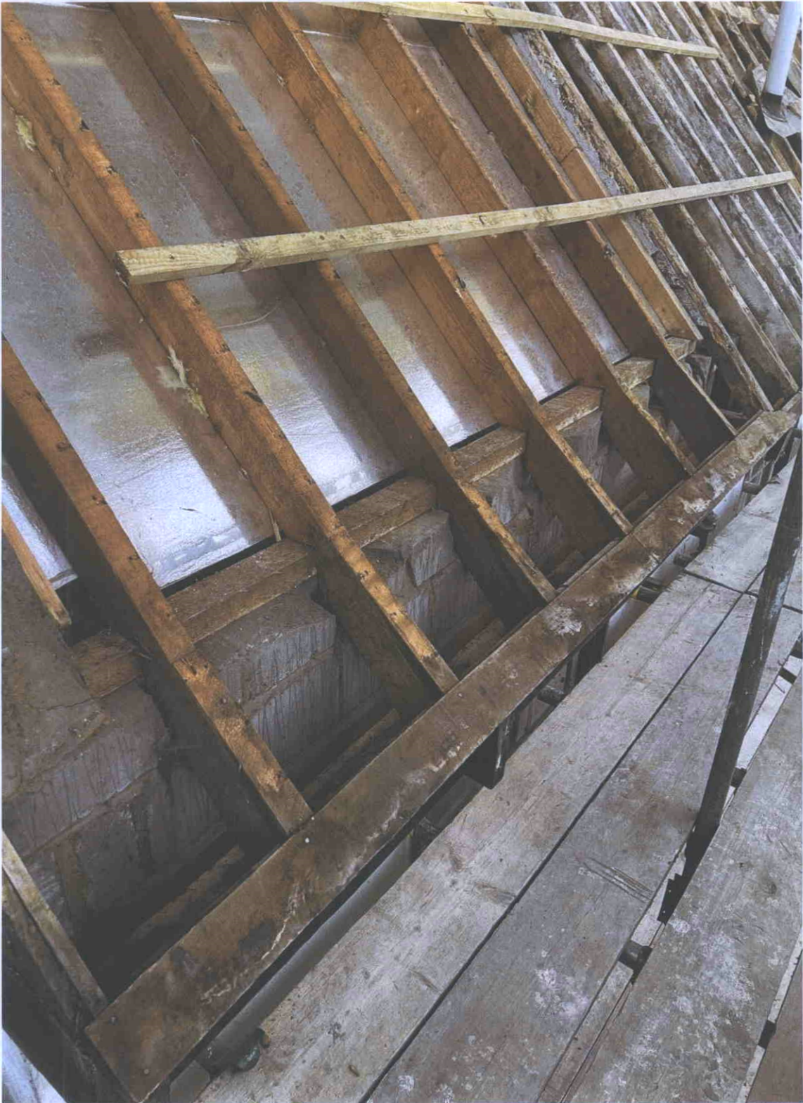
The bay 6 C20 roof slope on the north elevation (east end)
