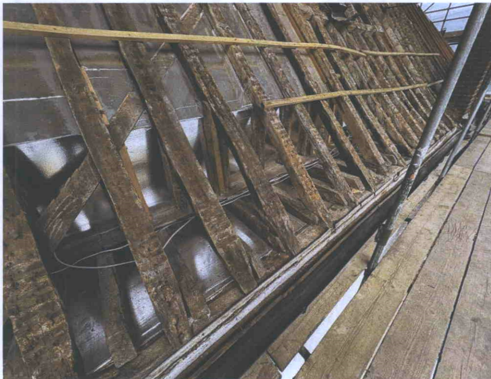
The south elevation roof slope showing short joist ends; at bay 3 at the left of the photograph and bay 4 to the right of the photograph.
