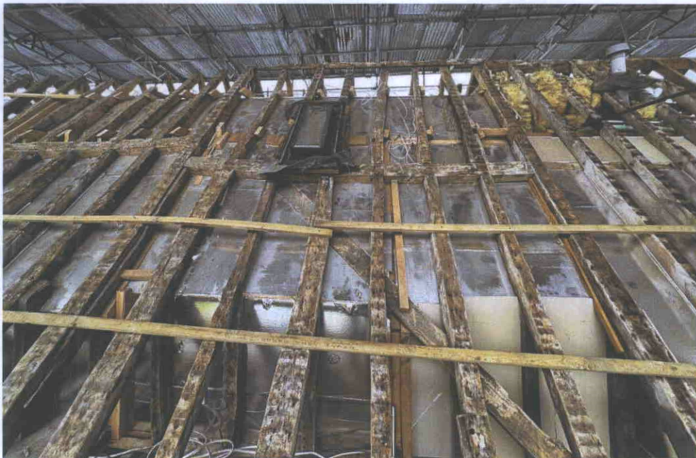
The south elevation roof slope of bay 3 shown on the left of the photograph; bay 4 centre of the photograph; and bay 5 shown to the right of the photograph.
