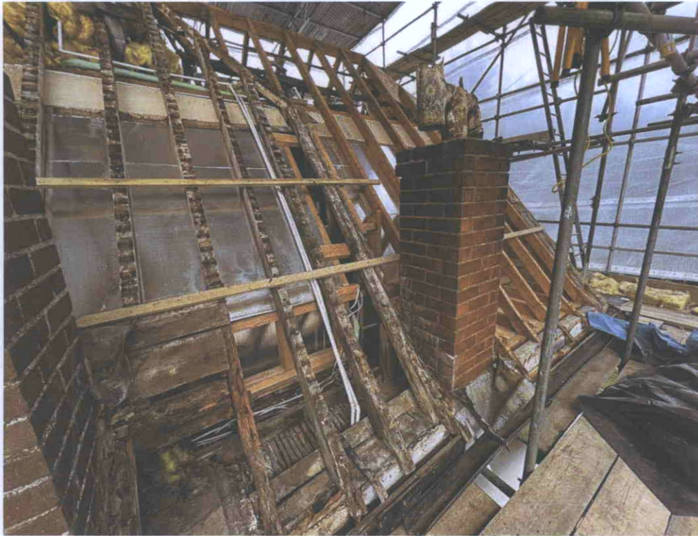
The bay 5 C19 roof slope on the south elevation and bay 6 C20 roof slope shown to the right of the photograph.
