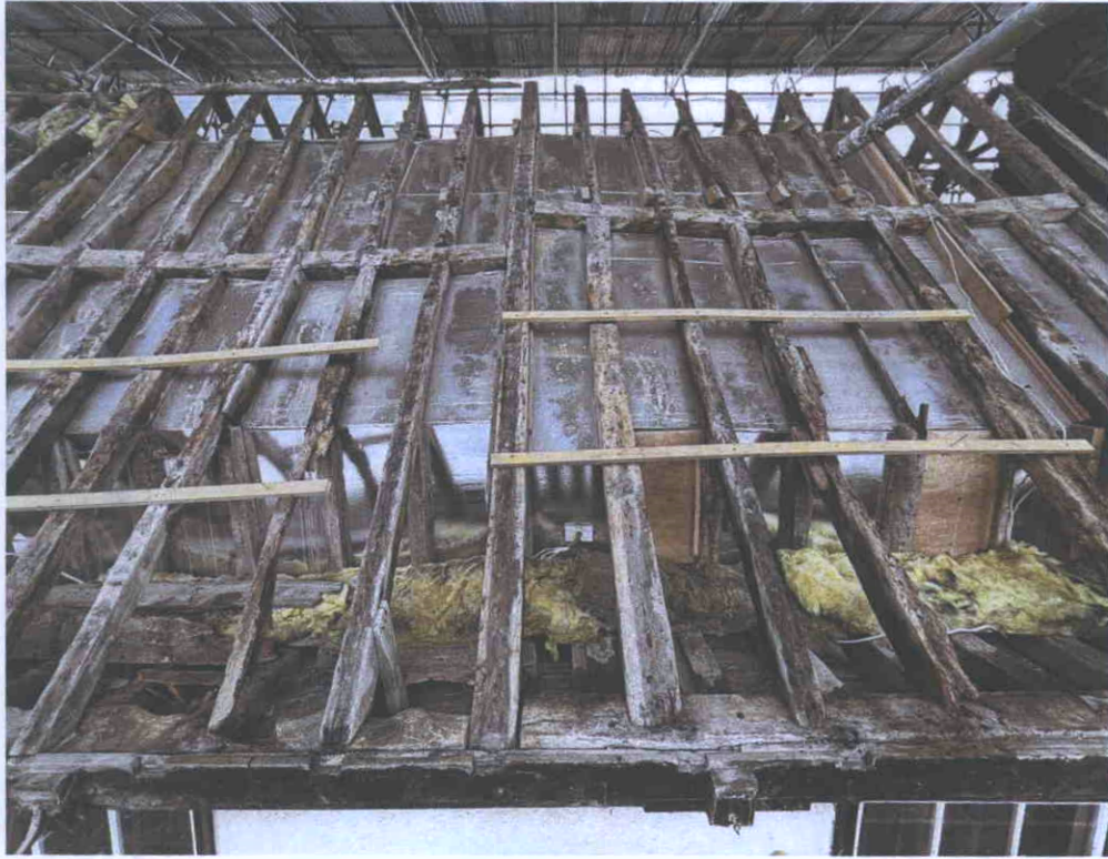
Bay 4 (L/H side) and Bay 3 (R/H side) north
