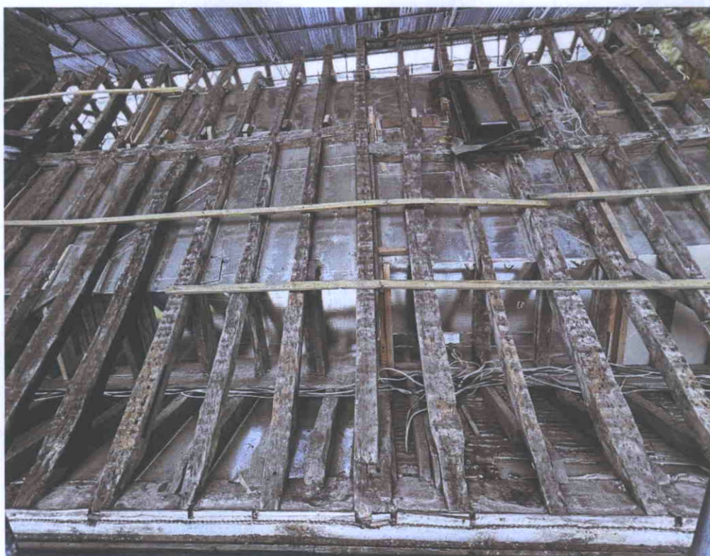
Bay 3 (L/H side) Bay 4 (R/H side) south
