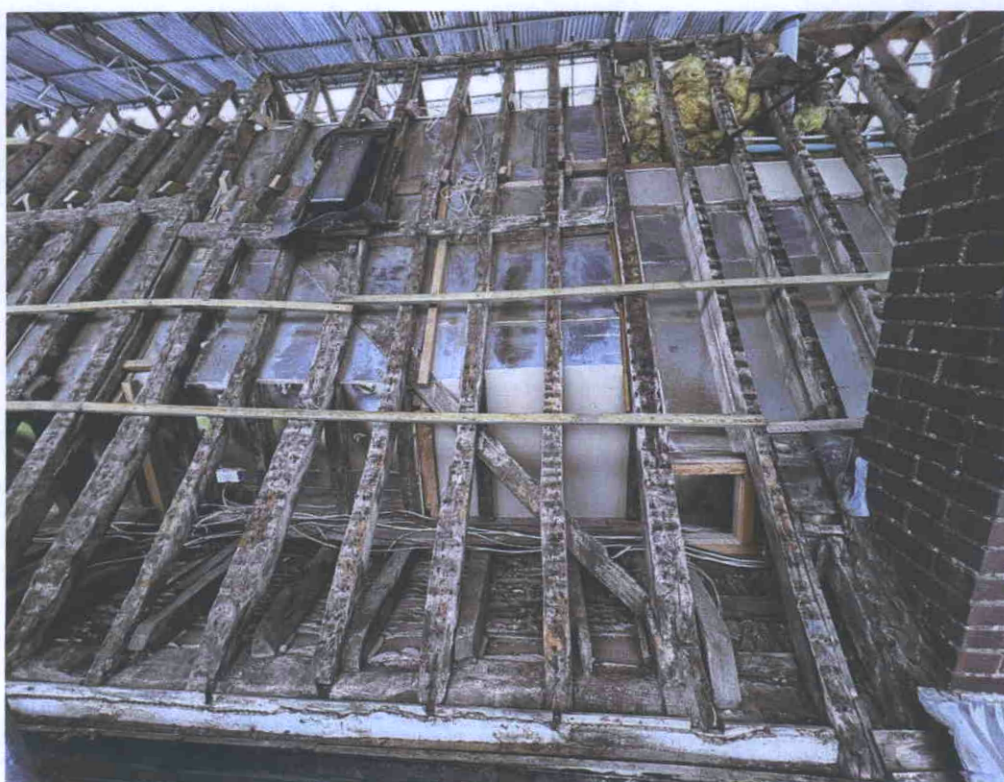
Bay 3 (L/H side) Bay 4 (centre) and Bay 5 (R/H side) south
