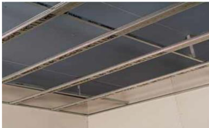
Figure 8 - Typical independent MF ceiling
