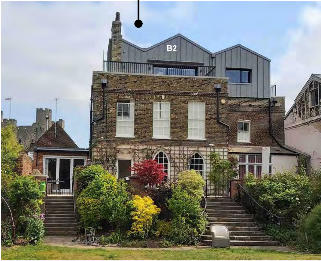
Fitch House with zinc clad extension to Grade II Listed house in Rochester by Clay Architecture
