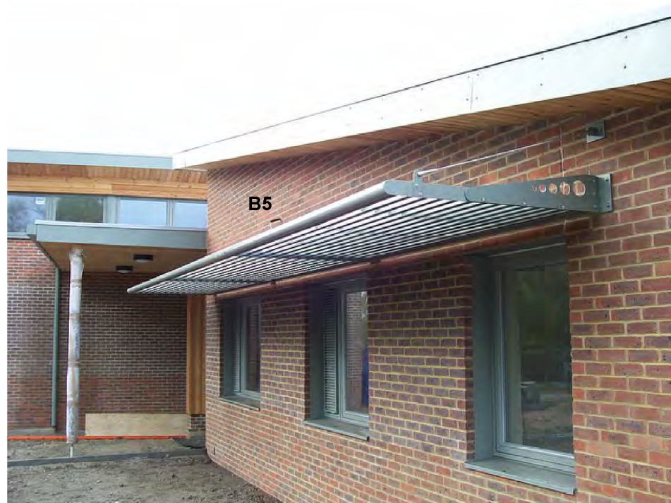
Brise soleil: polyester powder-coated aluminium with an elliptical profile.
