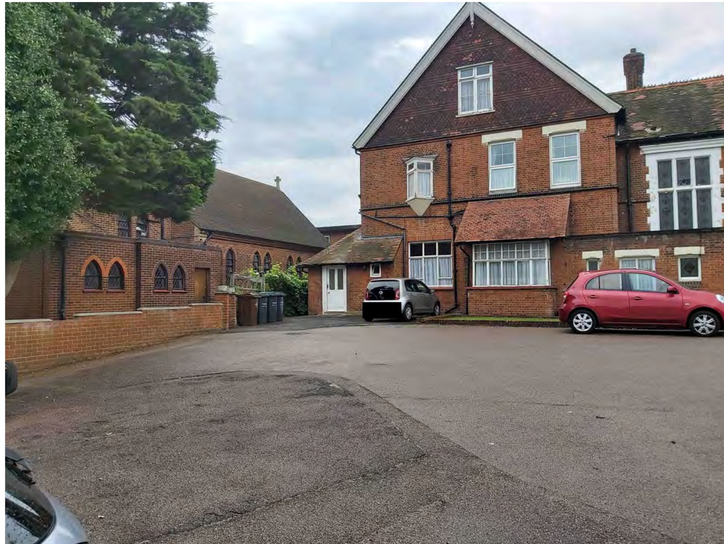
Front elevation with the chapel to the left
