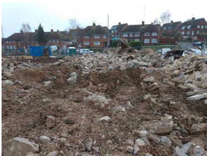
Plate 19: Block 3 slab removal.
