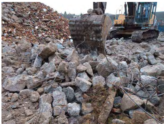
Plate 14: Block 4 slab removal.
