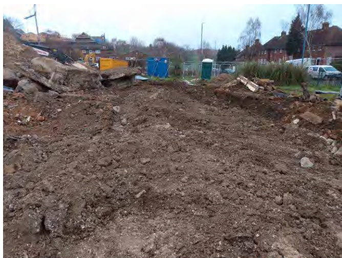
Plate 2: Block 3 slab removal.
