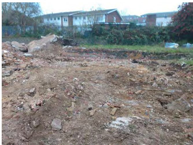
Plate 2: Block 1 slab removal.
