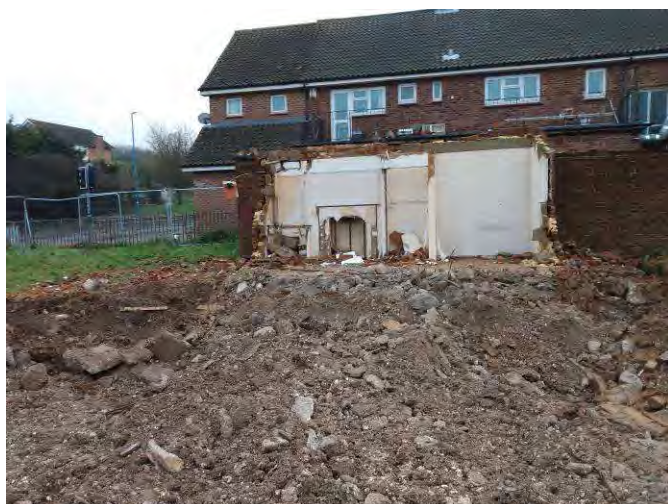
Plate 4: Block 3 slab removal and garage demolition south.
