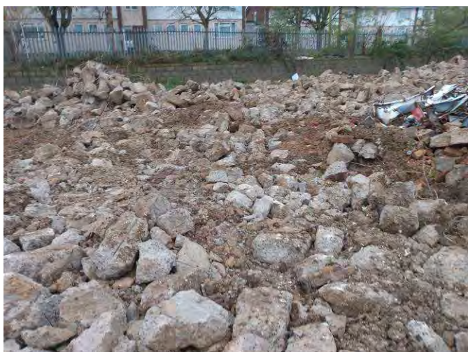
Plate 21: Block 2 slab removal.
