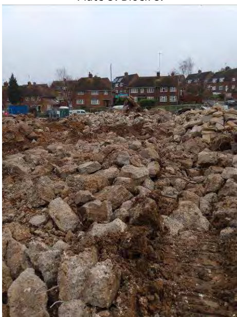
Plate 5: Block 3 slab removal.
