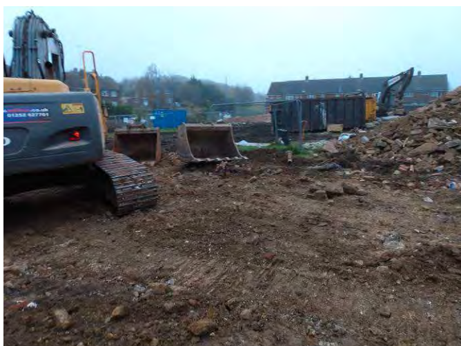
Plate 3: Block 1 slab removal.
