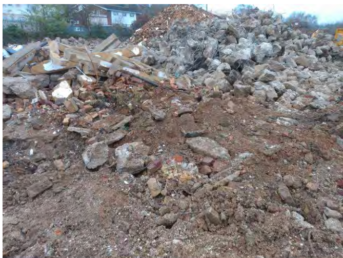
Plate 23: Block 2 slab removal.
