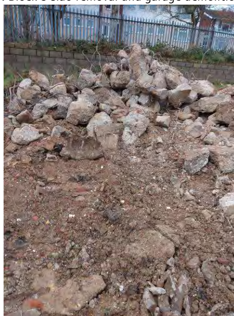
Plate 6: Block 3 slab removal.
