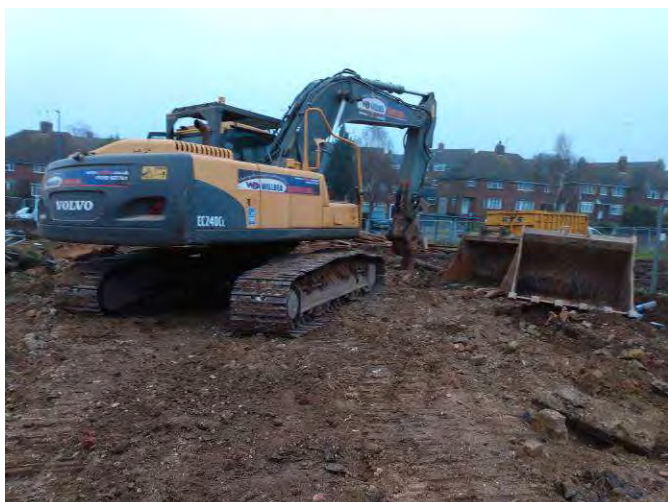
Plate 1: Block 1 slab removal.
