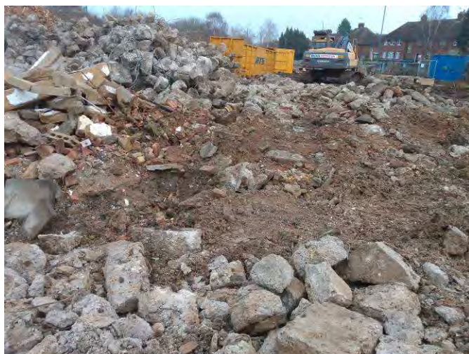
Plate 20: Block 3 slab removal.
