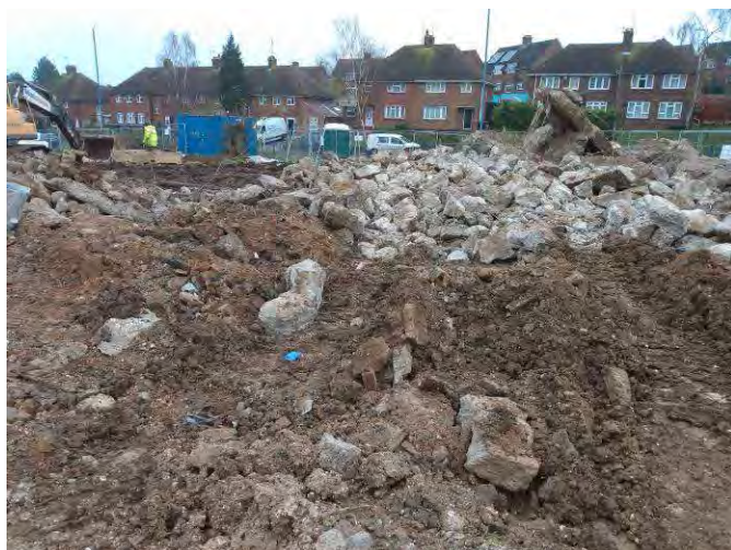
Plate 24: Block 2 slab removal.
