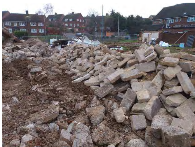
Plate 22: Block 2 slab removal.
