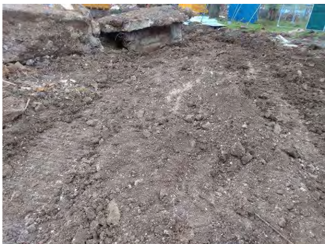
Plate 1: Block 3 slab removal.
