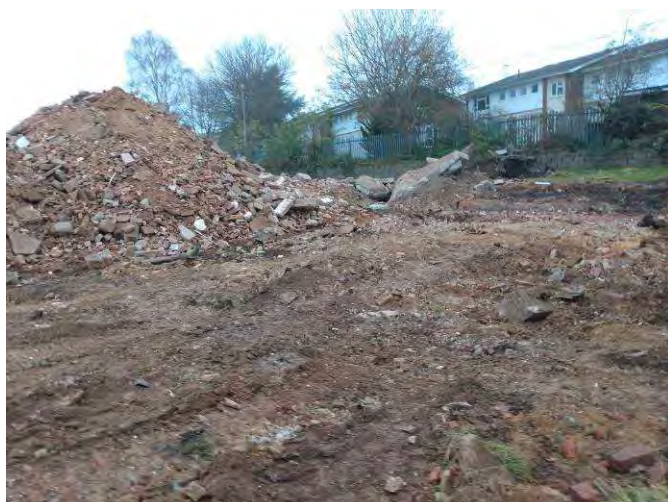
Plate 4: Block 1 slab removal.
