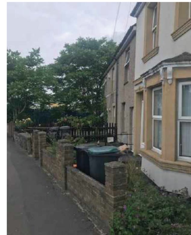
Photo 10: a small row of residential terrace houses located in the western corner of the site along Stonebridge Road.
