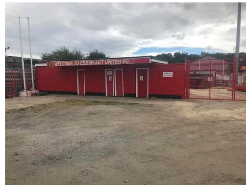
Photo 14: standing north-west of the Football ground looking west. Evidence of hydrocarbon spills on the gravelled ground which is used for vehicle parking.
