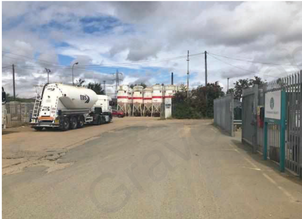
Photo 24: aggregate mix storage tanks associated with Britannia Aggregates looking north-west.
