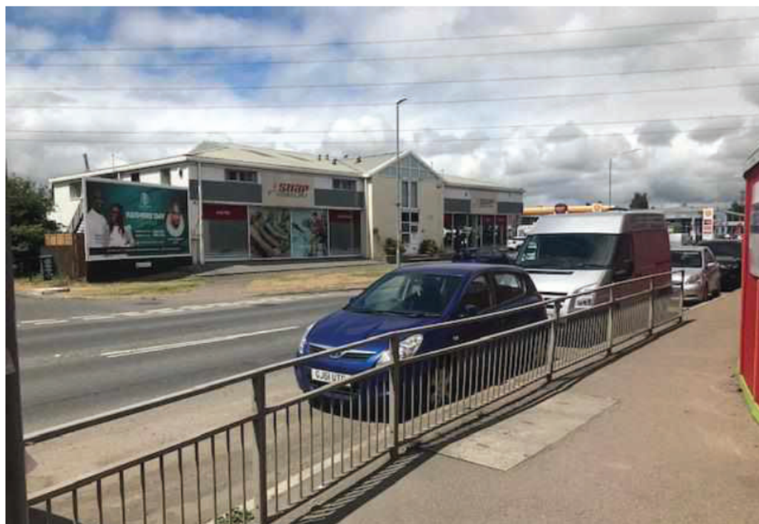
Photo 31: Ebbsfleet Fitness Centre located in the south-west of the site along Stonebridge Road.
