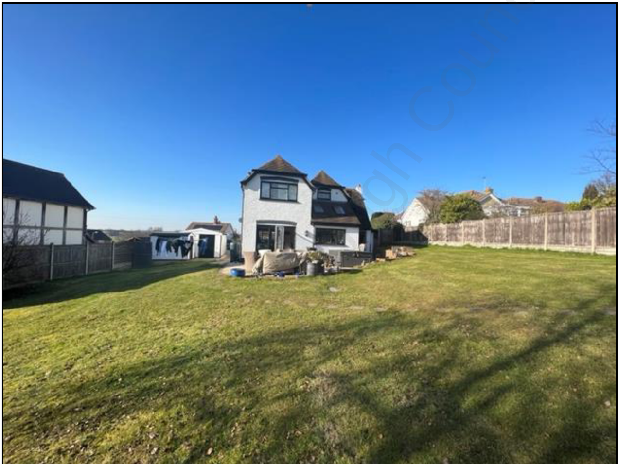
Photograph of the dwellinghouse taken from rear, showing relationship with adjoining neighbours.
