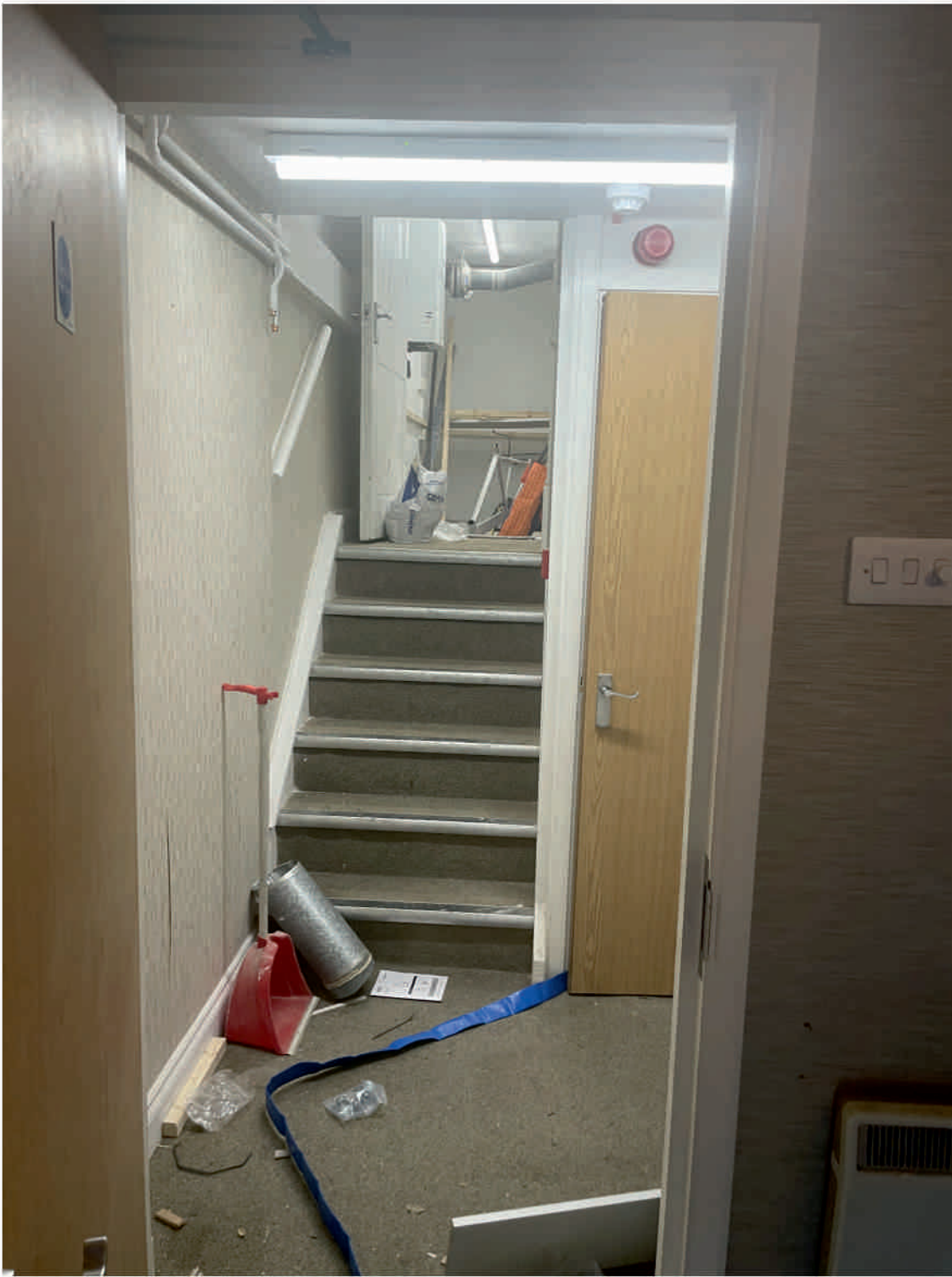
AREA 11 STAIRS - Looking from room 10 showing stair covered with nosings and carpet. Also shows door the lower cellar level no access. No original features except covered stair.
