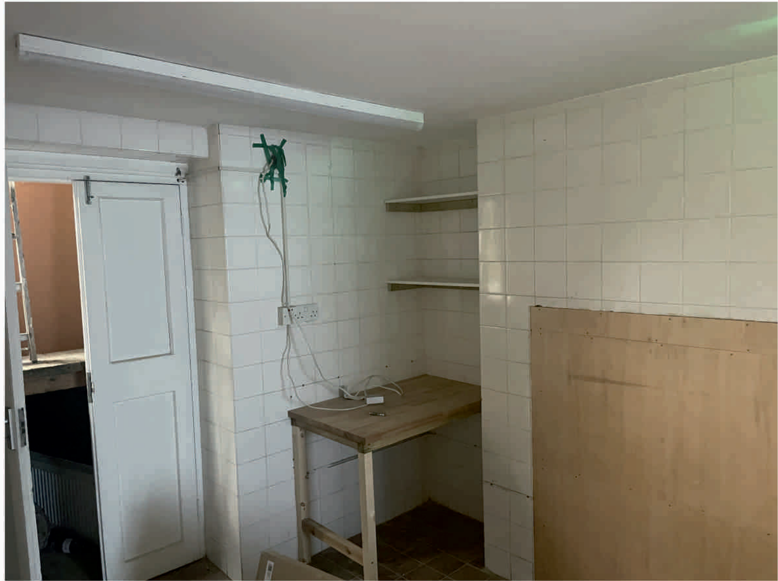
ROOM 12 - Facing double door to cellar flap recess noting ground floor level at half door height. No original features.
