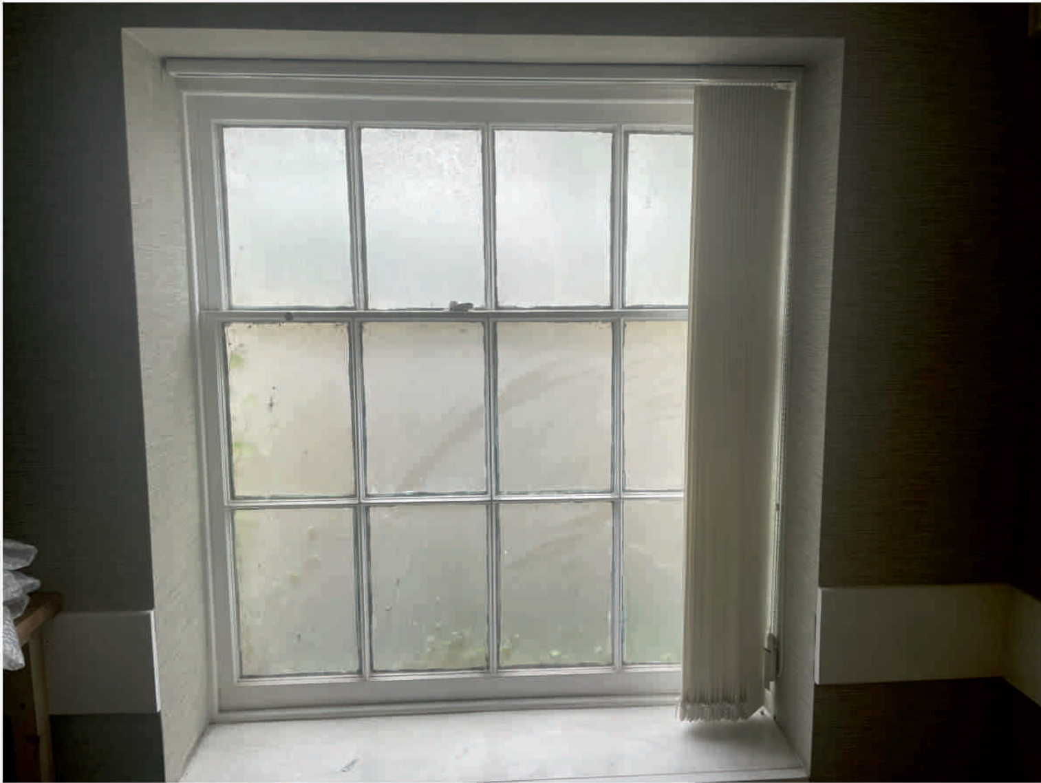
ROOM 13 - Photograph of original ash window in light well in good working order to be made good and retained incorporating new secondary glazing. No other original features.
