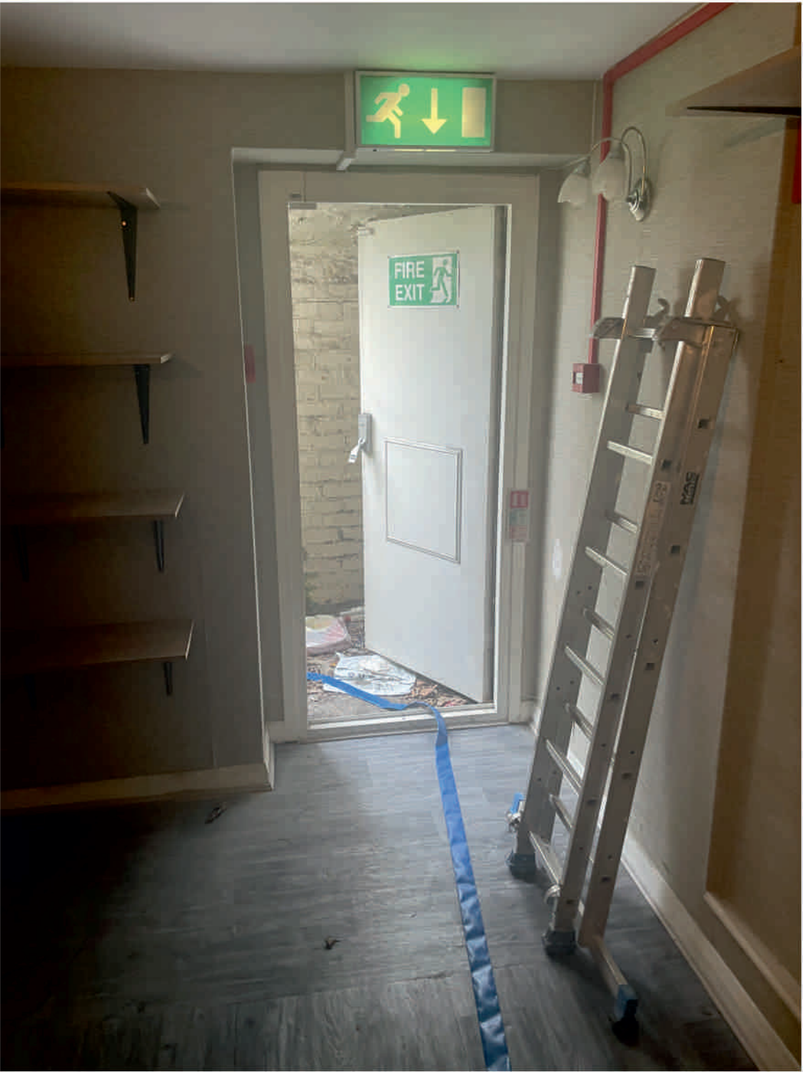
ROOM 10 - Facing toward fire exist door and external steps to footway under ground floor entrance steps. Partition wall to locked store is shown to the right. No original features.
