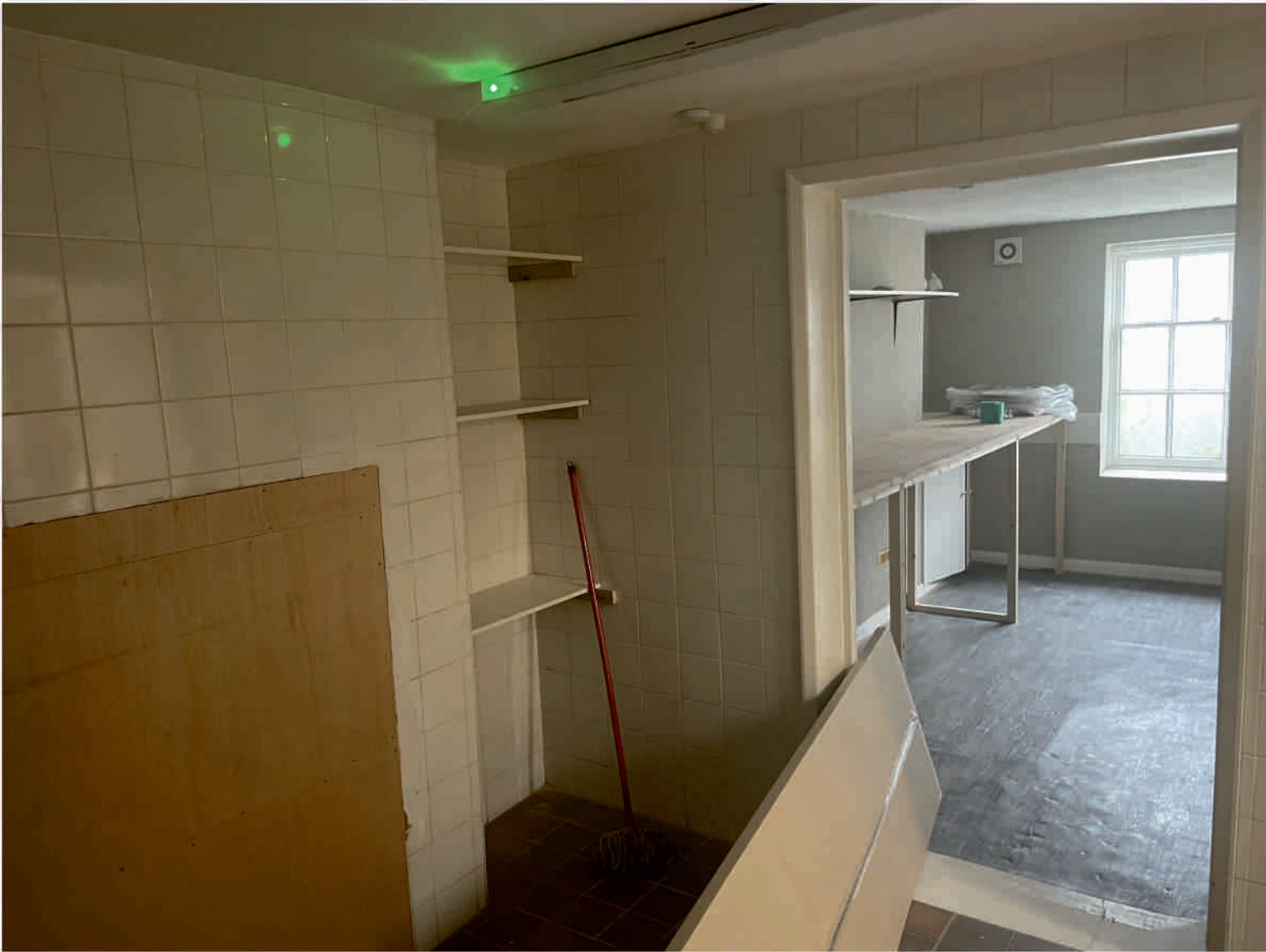
ROOM 12 - Facing light well window in room 13 through connecting double doors. No original features
