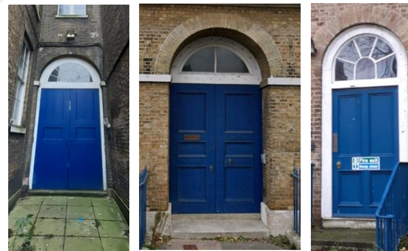
External doors to be refurbished and retained.
