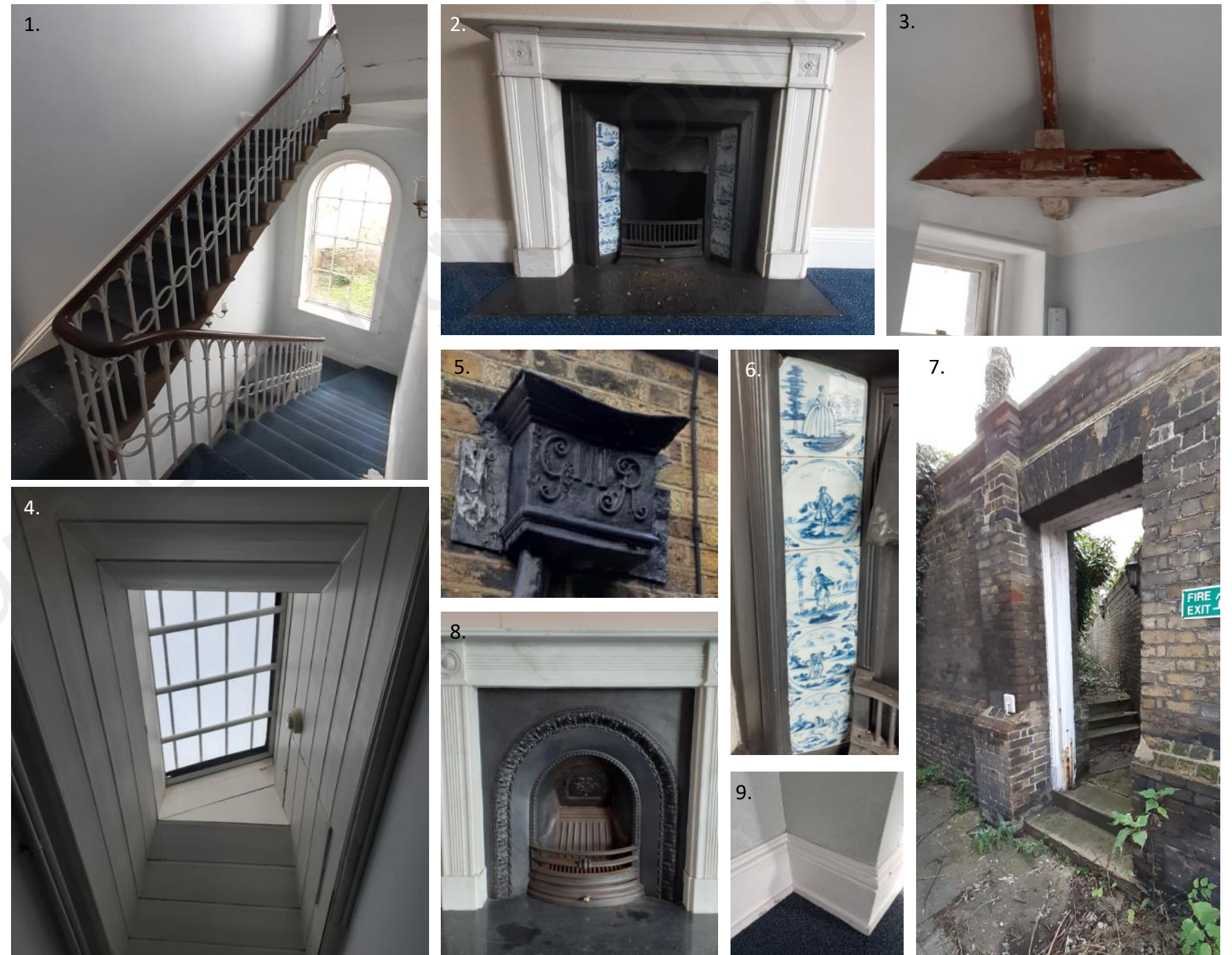
1. Original staircase designed by Robert Adams. 2. Original fireplace 3. Exposed Timber Roof Beam 4. Original Skylight 5. Cast Iron Rainwater Hopper 6. Tiled insert from original fireplace 7. Spine Wall with original opening. 8. Original Fireplace 9. Original Skirting
