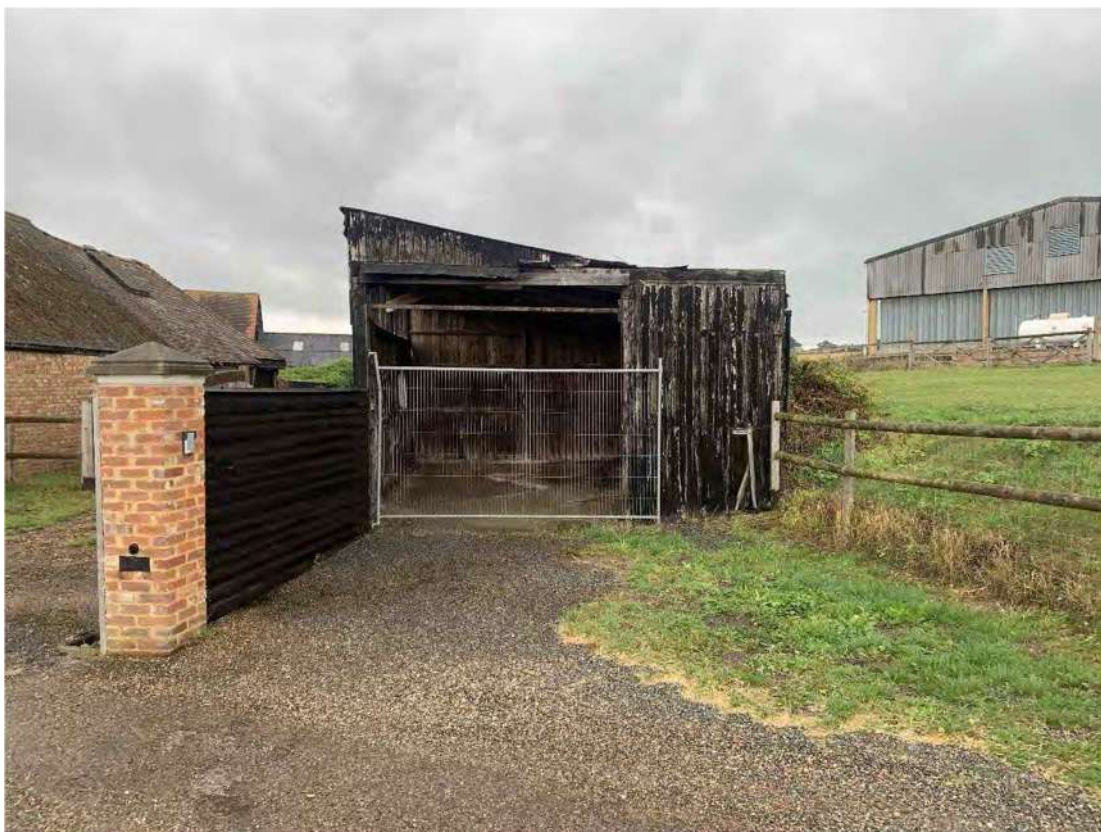
Plate 37: Building 13 looking south-east
