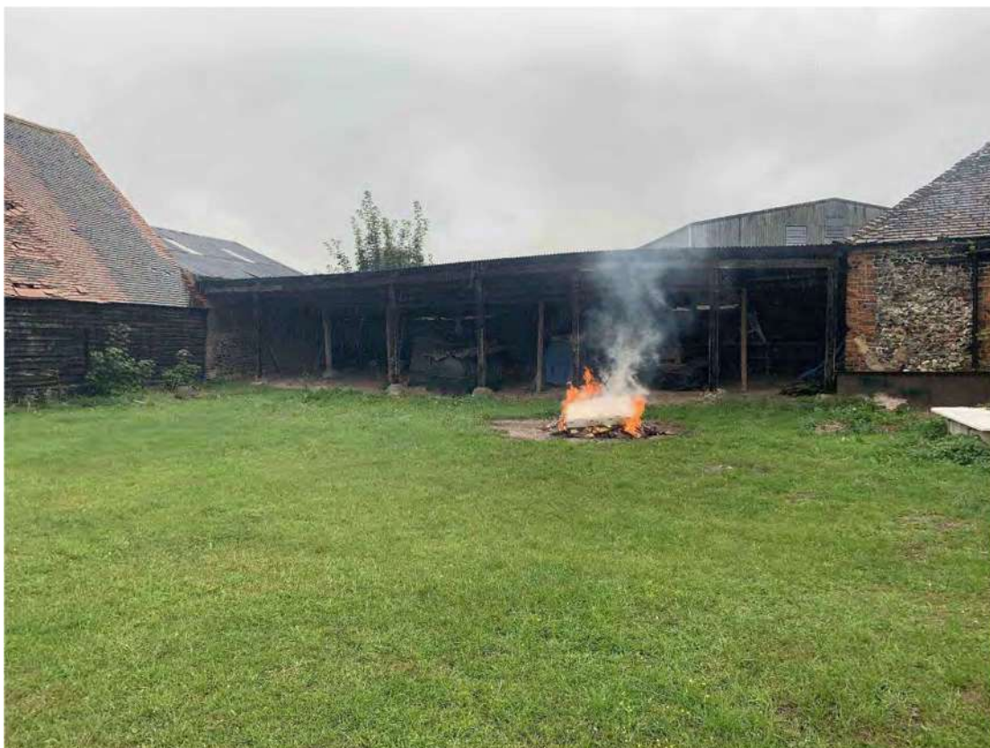
Plate 23: Building 9 looking south
