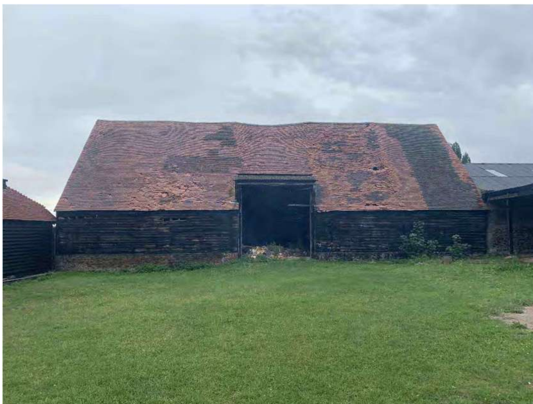
Plate 12: Building 5 looking south-east
