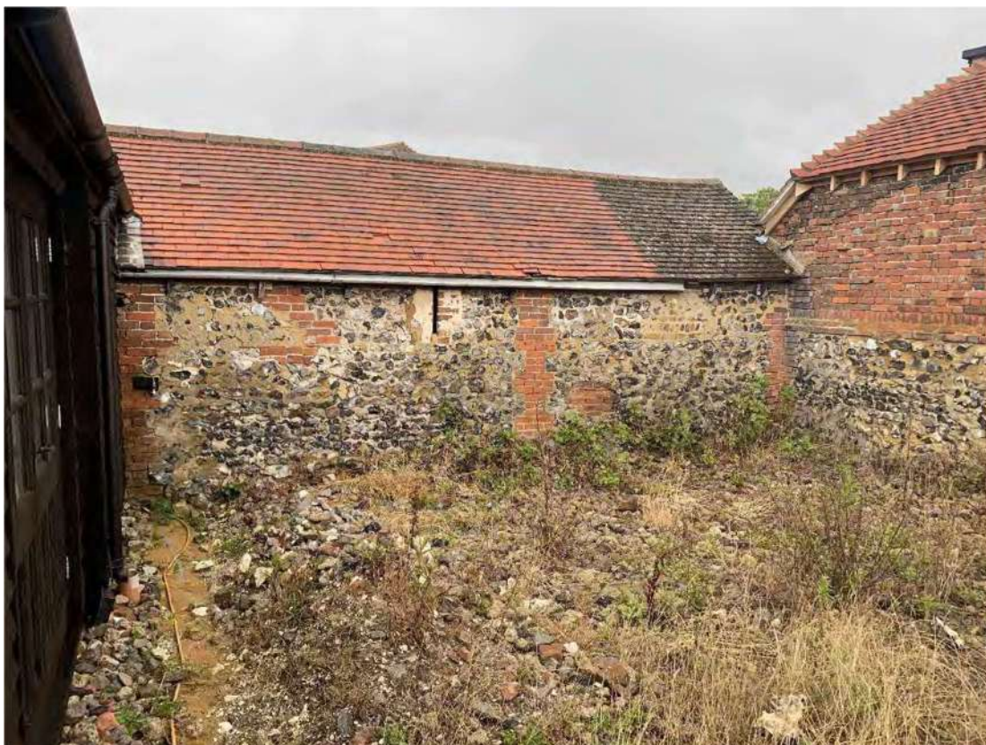
Plate 45: Building 15 looking north-east
