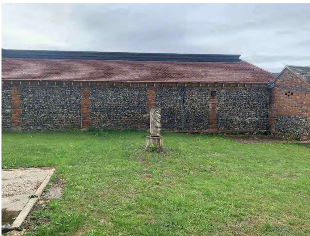
Plate 42: Building 14 looking south-west
