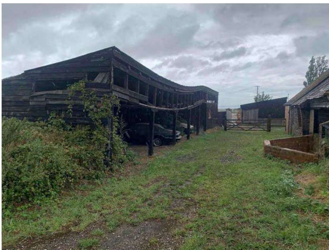
Plate 38: Building 13 looking west
