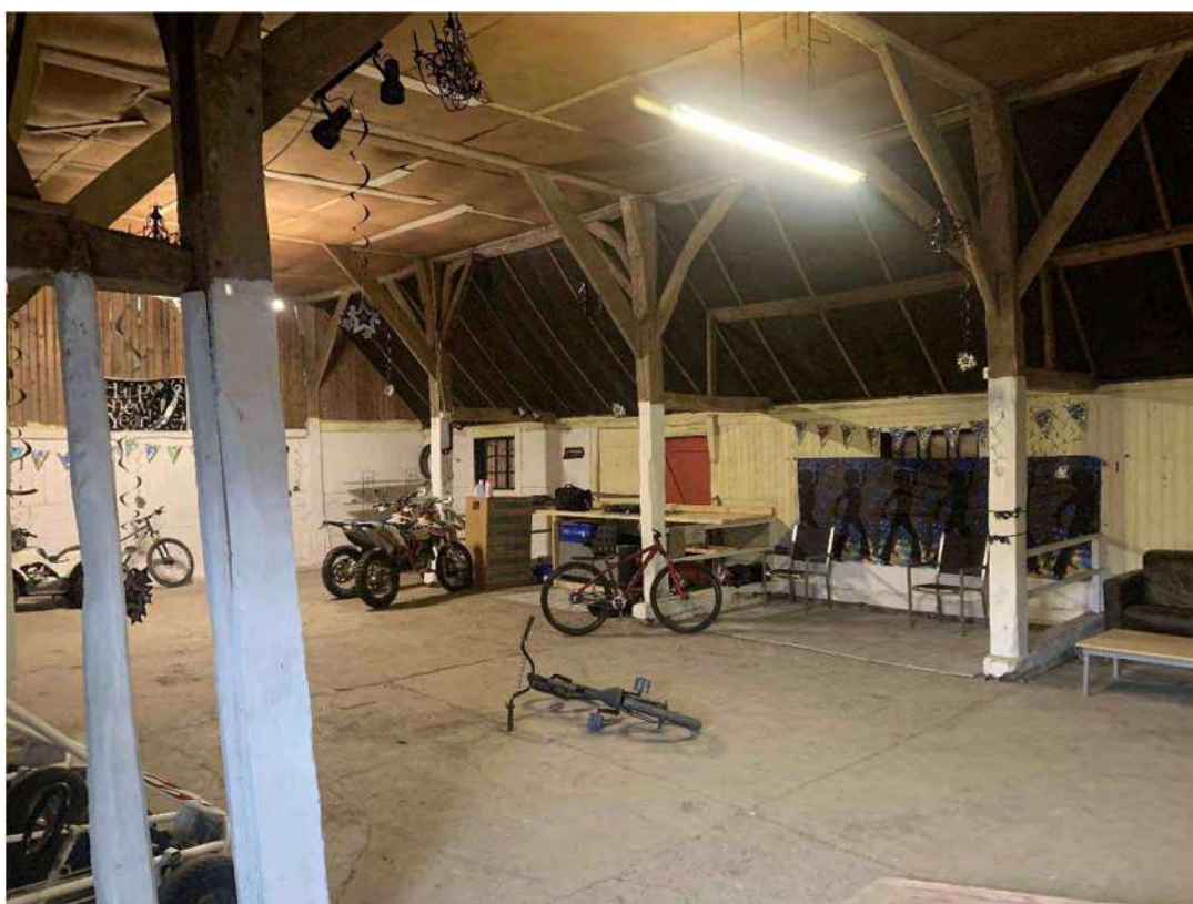
Plate 6: Interior of building 2 looking north-west
