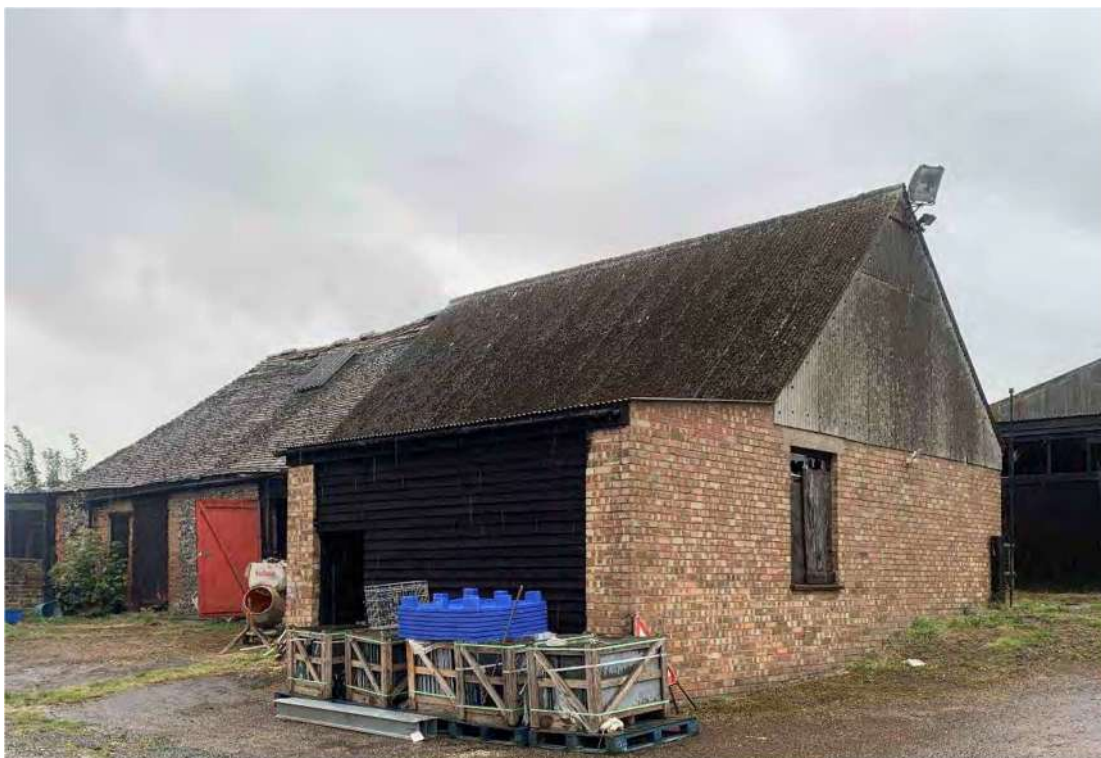
Plate 25: Building 10 looking south
