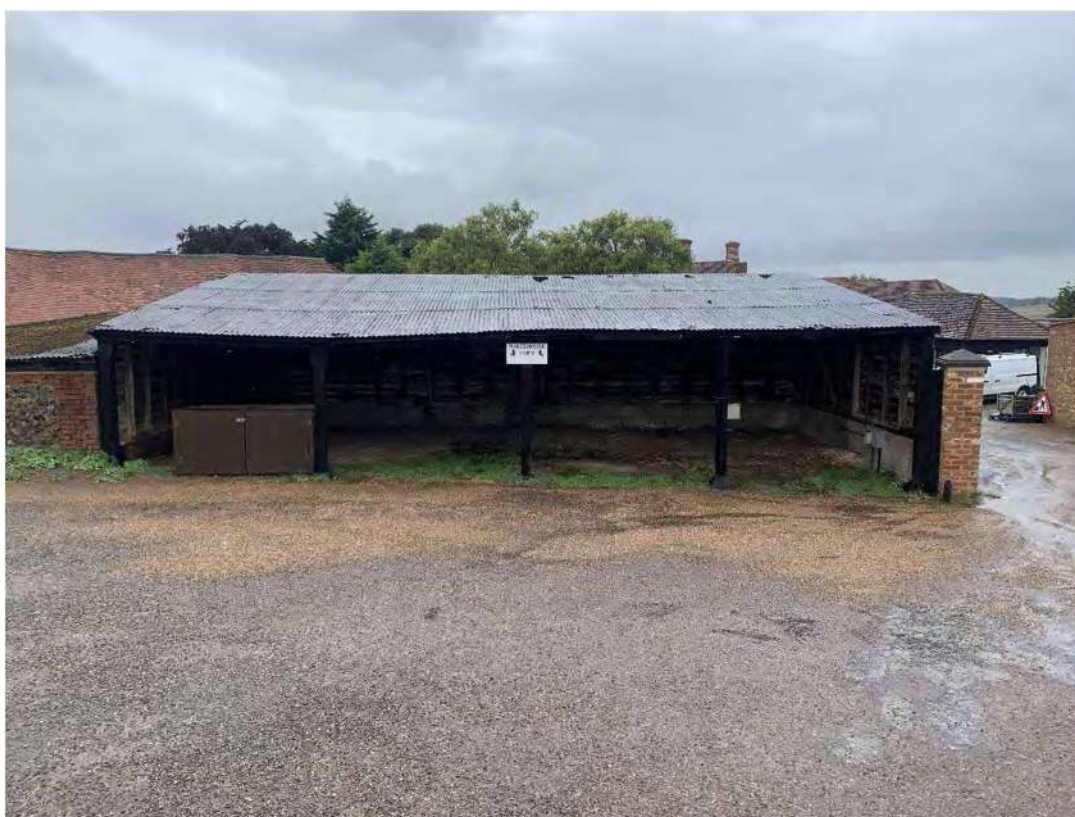
Plate 32: Building 11 looking north-east
