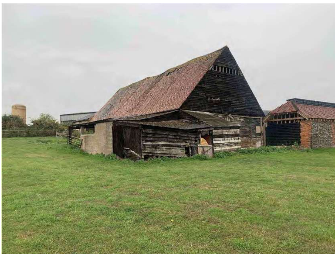
Plate 20: Building 7 looking south-west
