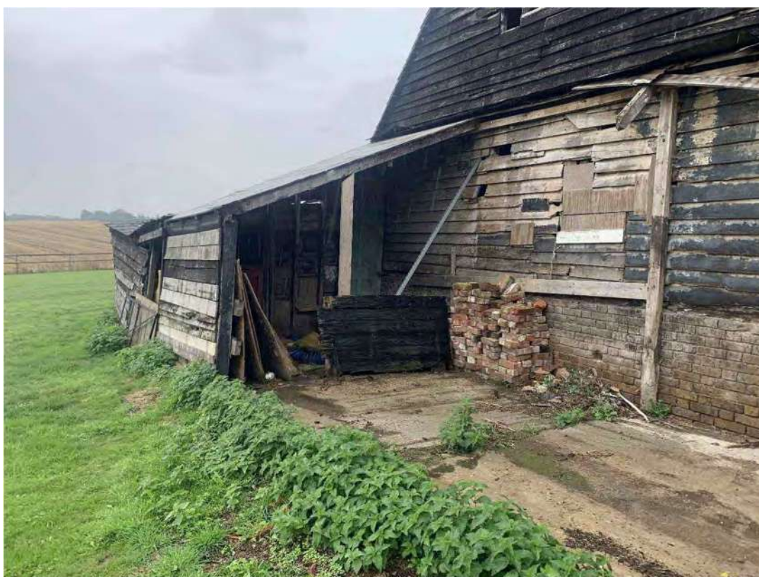
Plate 18: Building 6 looking south
