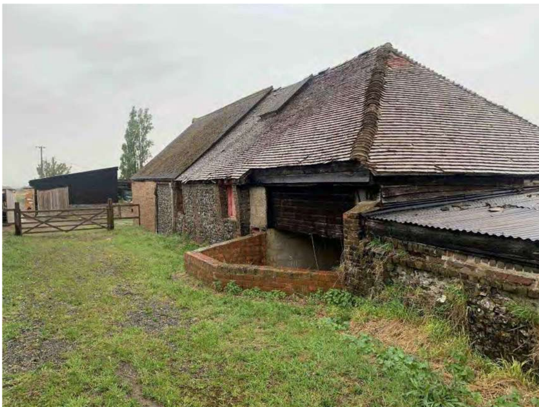
Plate 27: Building 10 looking north
