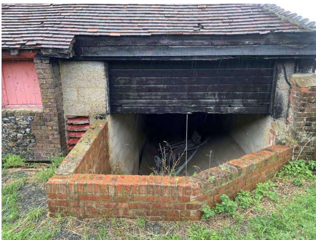
Plate 28: Detail of hopper at rear of building 10
