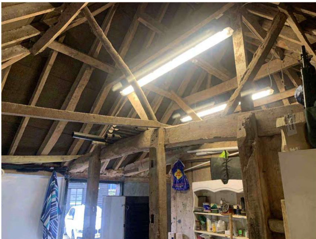
Plate 11: Interior of building 3 looking north-east
