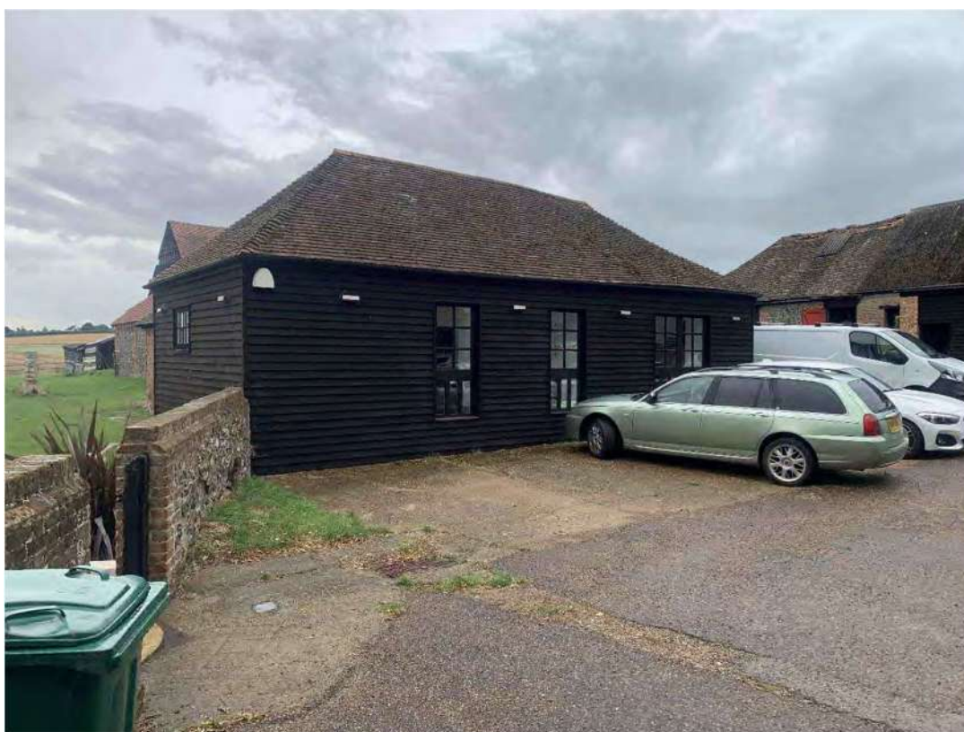
Plate 12: Building 4 looking south-east
