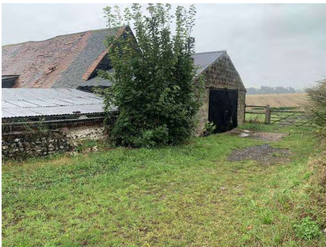
Plate 22: Building 8 looking south-east
