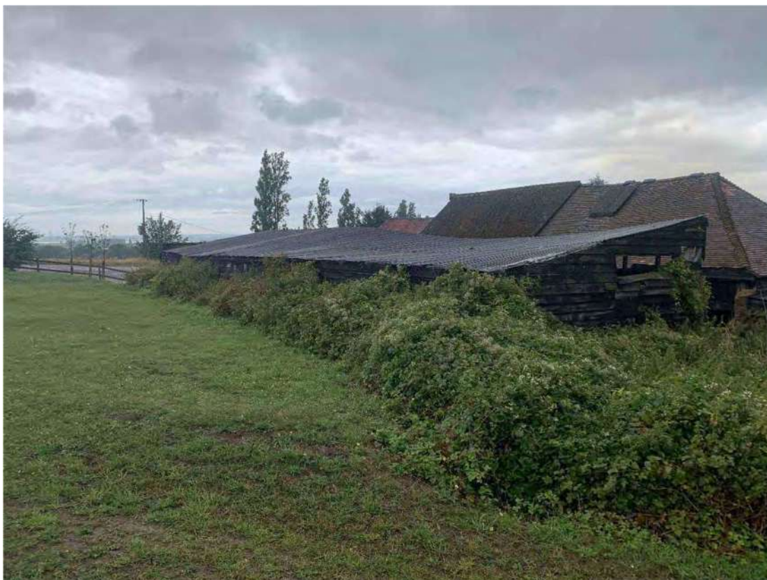
Plate 39: Building 13 looking north-west
