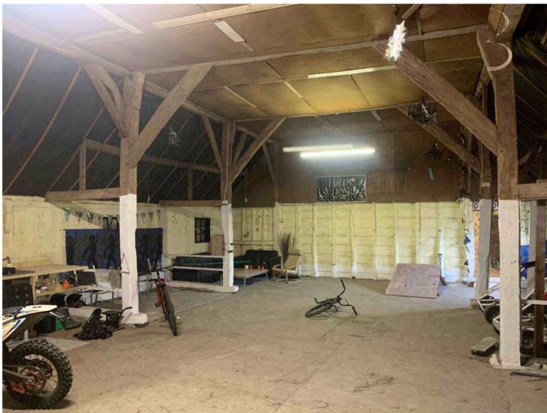
Plate 5: Interior of building 2 looking north-east
