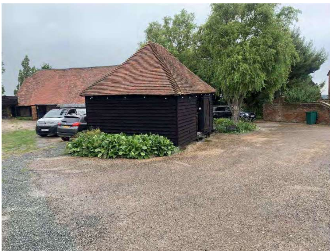
Plate 10: Building 3 looking north
