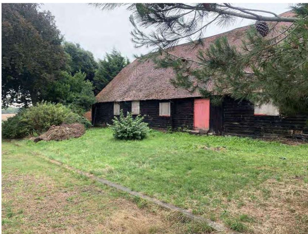
Plate 4: Building 2 looking south-east
