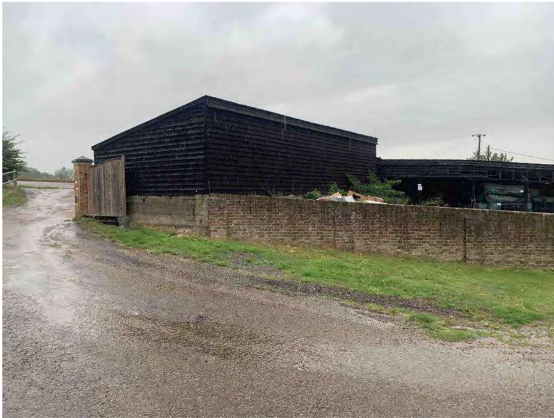
Plate 33: Building 11 looking west
