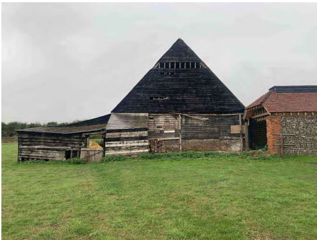
Plate 17: Building 6 looking south-west
