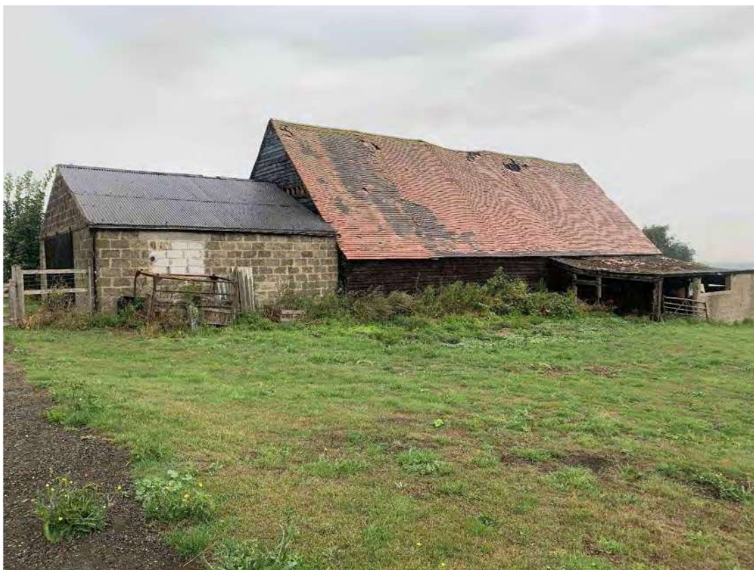
Plate 19: Building 7 and 8 looking north
