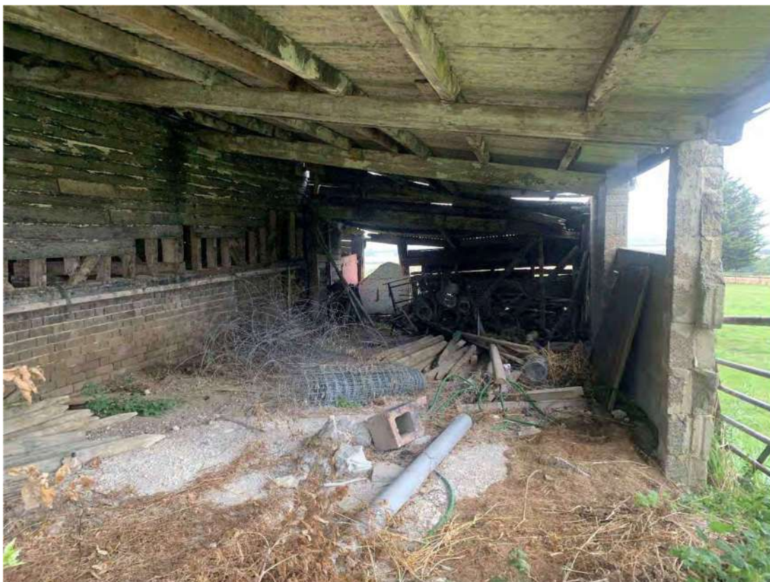
Plate 21: Interior of building 7 looking north-east
