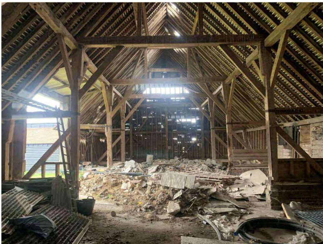
Plate 15: Interior of building 5 looking north-east
