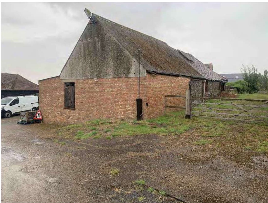
Plate 29: Building 10 looking east
