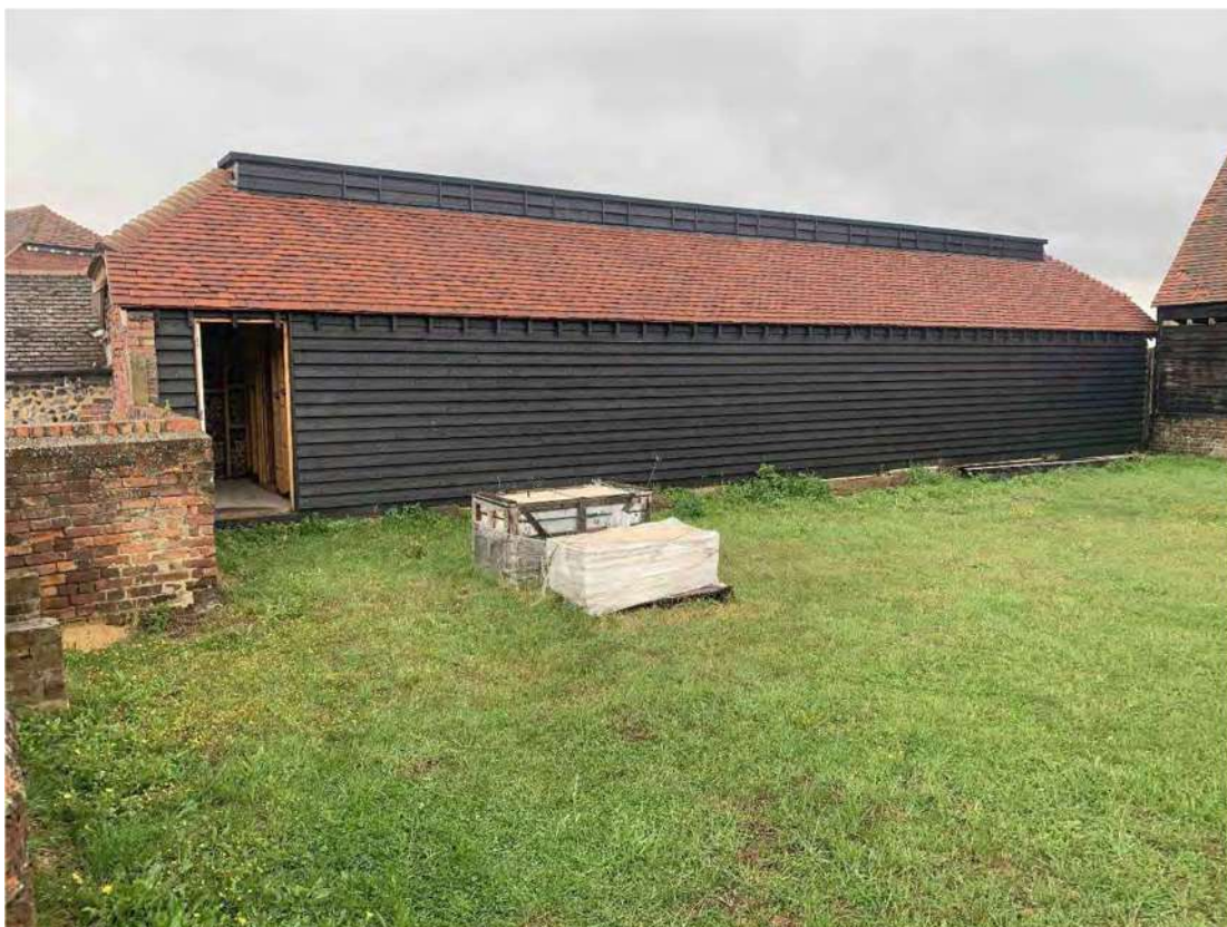
Plate 41: Building 14 looking east
