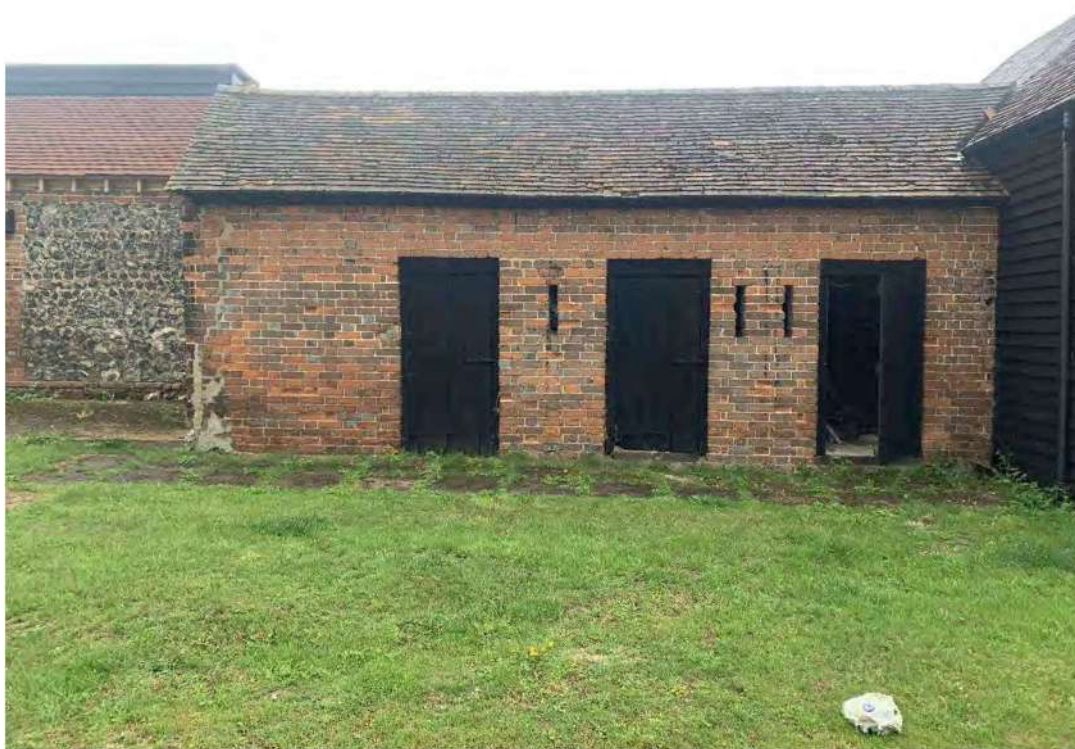
Plate 44: Building 15 looking south-west
