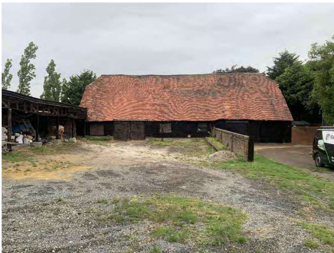
Plate 2: Building 2 looking north
