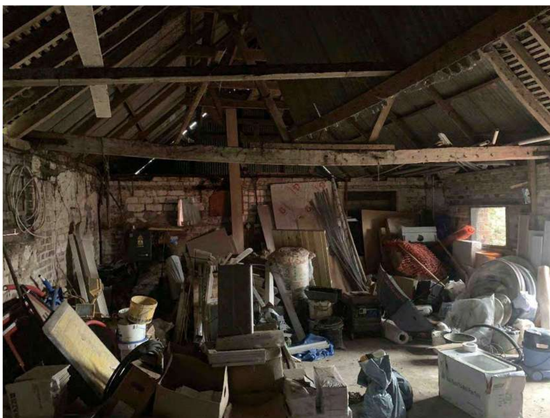
Plate 30: Interior of building 10 looking north-west
