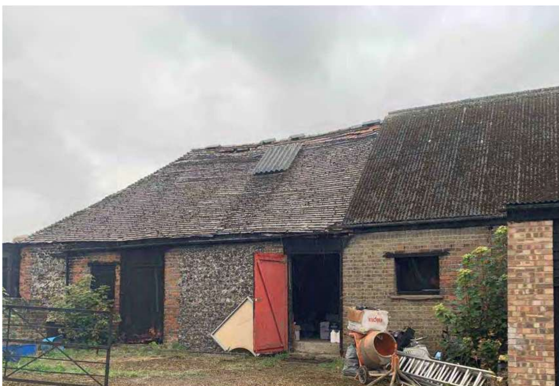
Plate 26: Building 10 looking south-west
