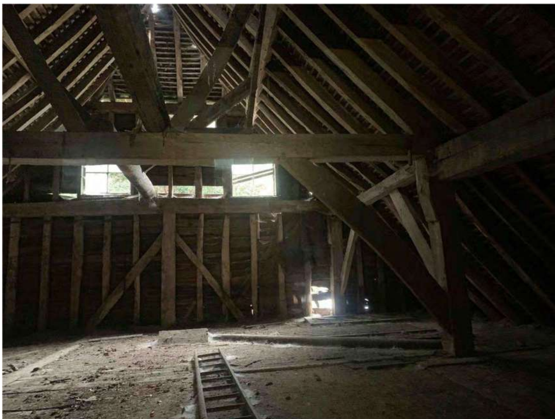
Plate 9: Roof structure of building 2 looking east
