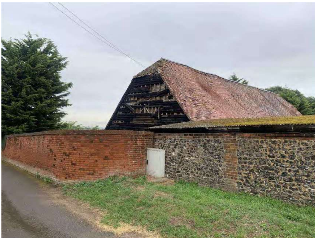
Plate 3: Building 2 looking north-east
