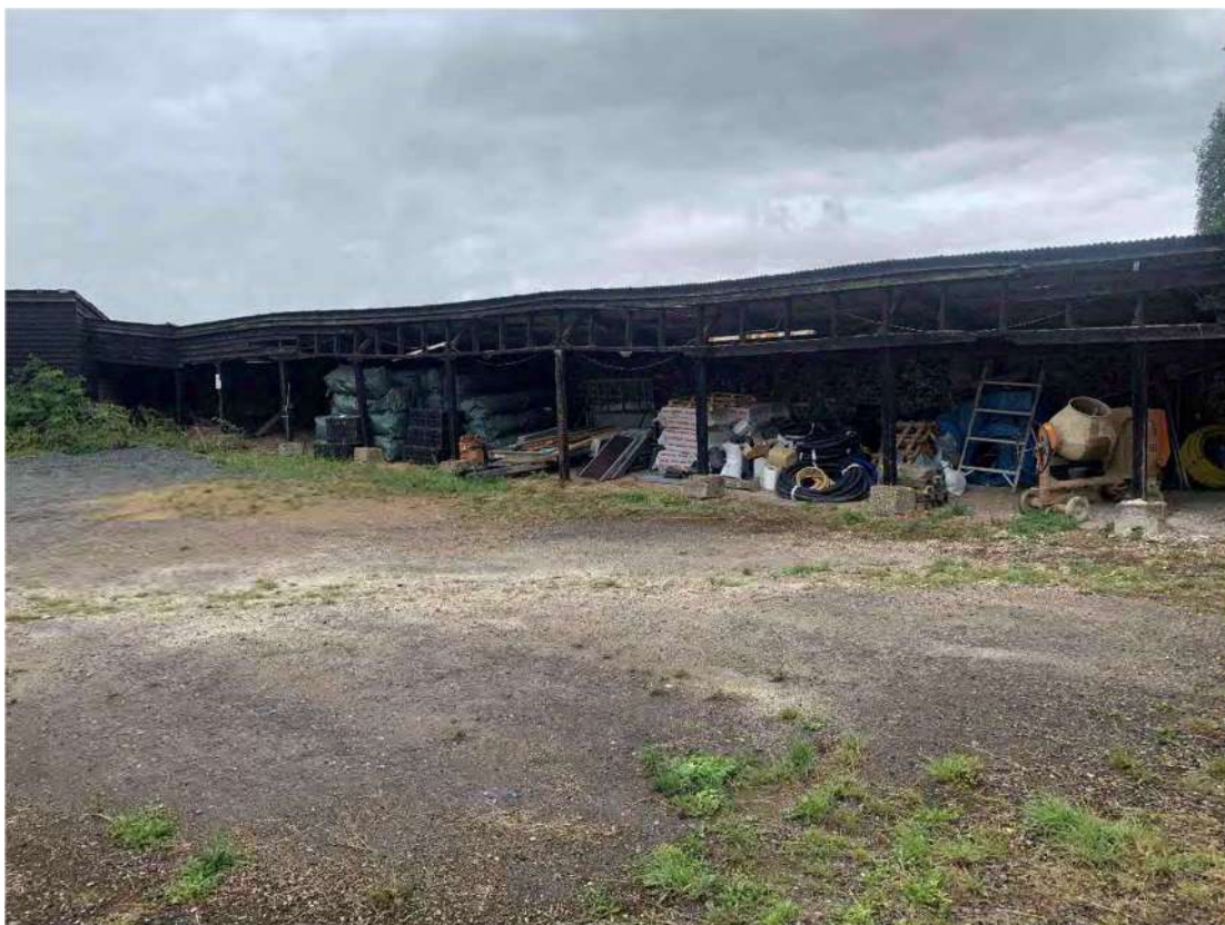
Plate 35: Building 12 looking south-west
