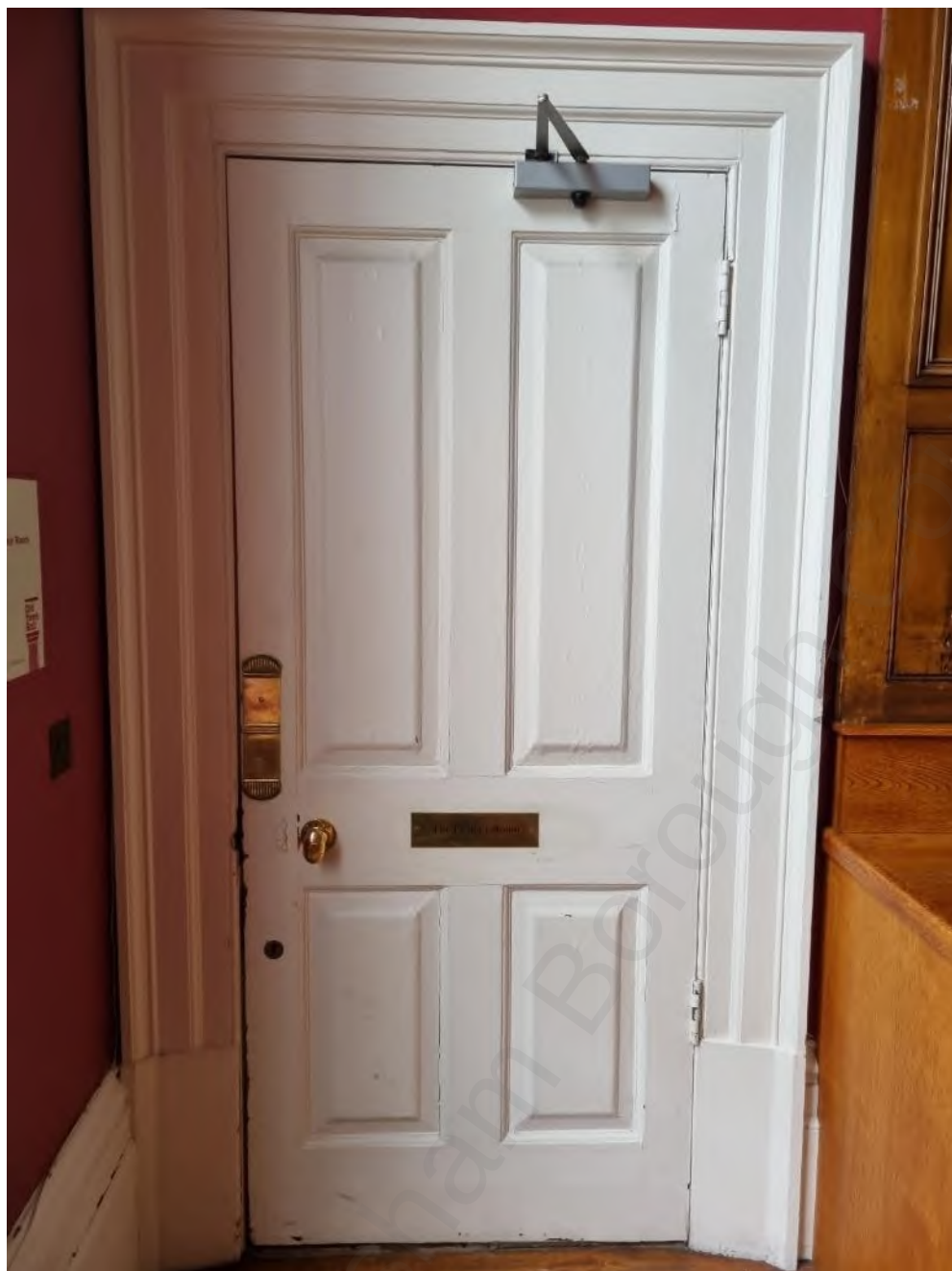
Photo 23: Door to Old Parlour Room
