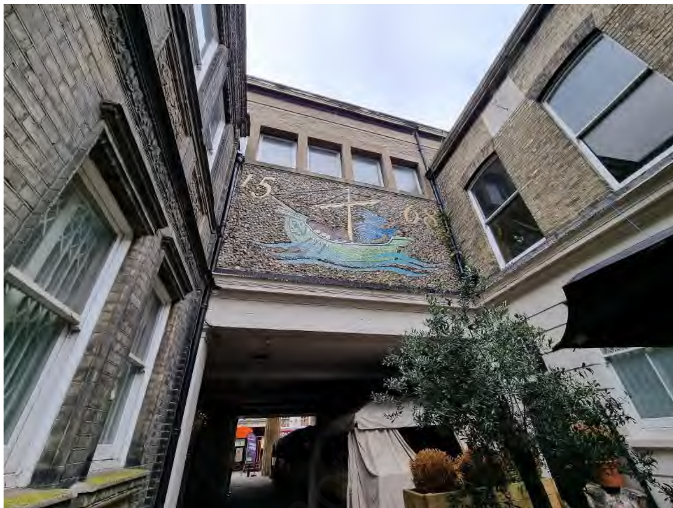
Photo 4: Detail image of modern mosaic covering eastern elevation at rear of original west range of Old Town Hall
