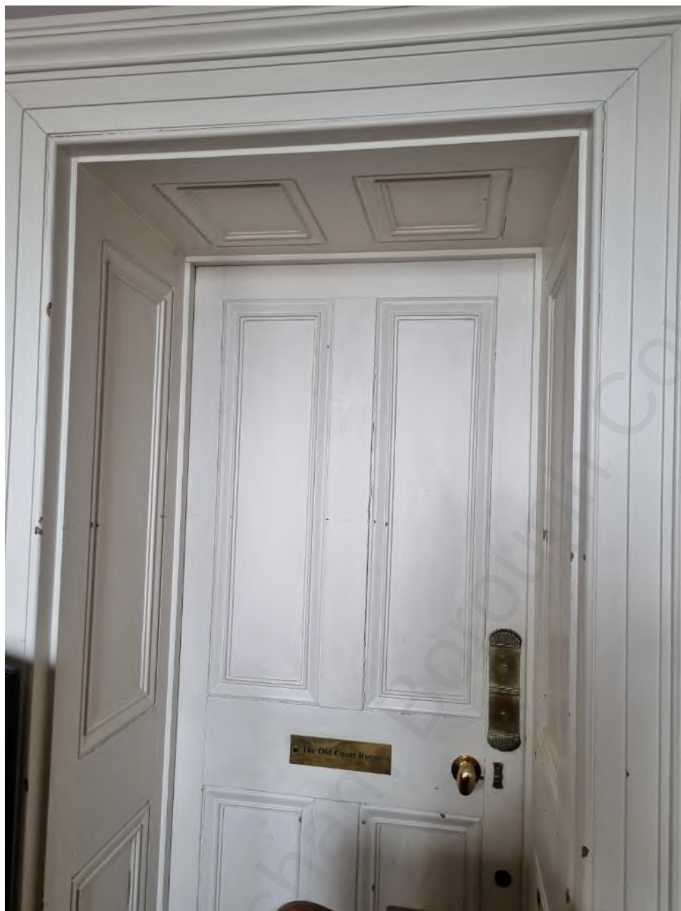
Photo 20: Existing door to Old Court Room
