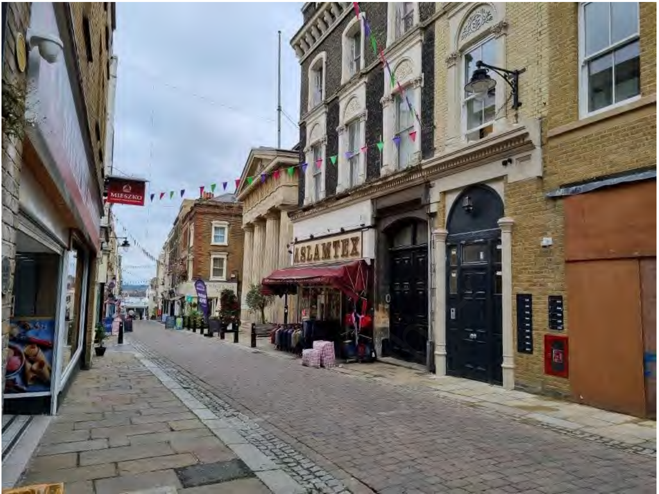
Photo 2: Oblique view across western frontage of Old Town Hall showing restricted visibility at short range
