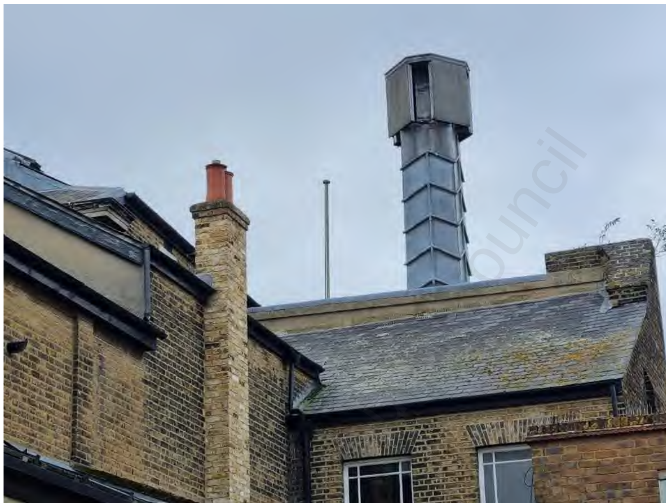
Photo 9: General view of roof condition, view to south west
