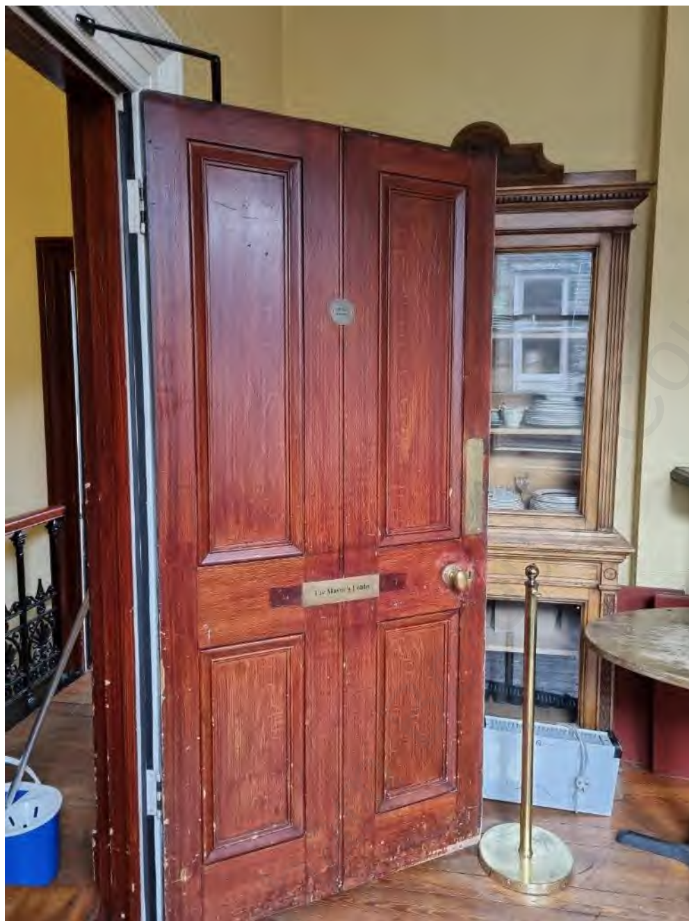
Photo 24: Existing door to Mayor's Lobby
