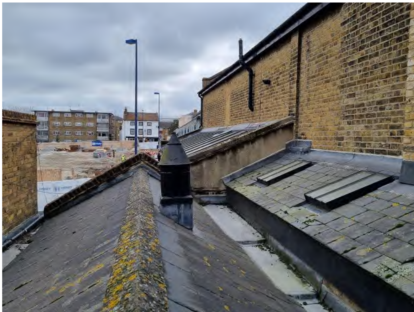
Photo 8: Indicative view of existing roof condition, view to east
