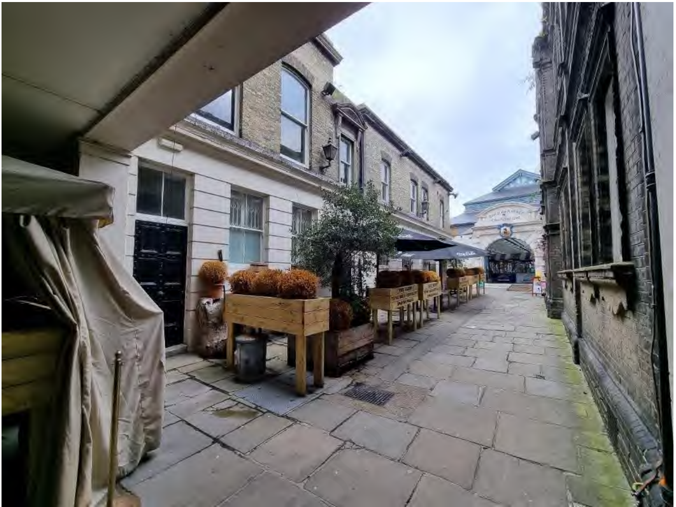
Figure 3: General view of the passageway between the rear wings of Gravesend Old Town Hall, facing east
