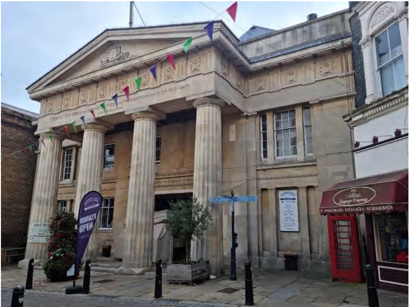
Photo 1: General view of Town Hall frontage taken from the High Street, facing north east
