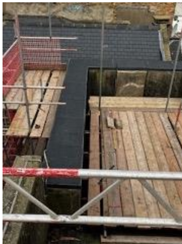
New parapet cappings
