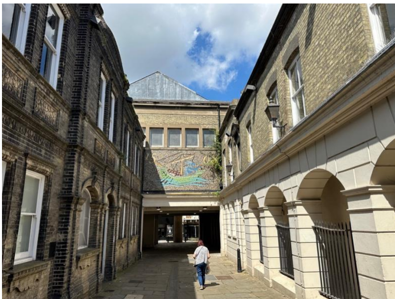
View of the passageway between the two wings of Gravesend Old Town Hall looking back towards the High Street
