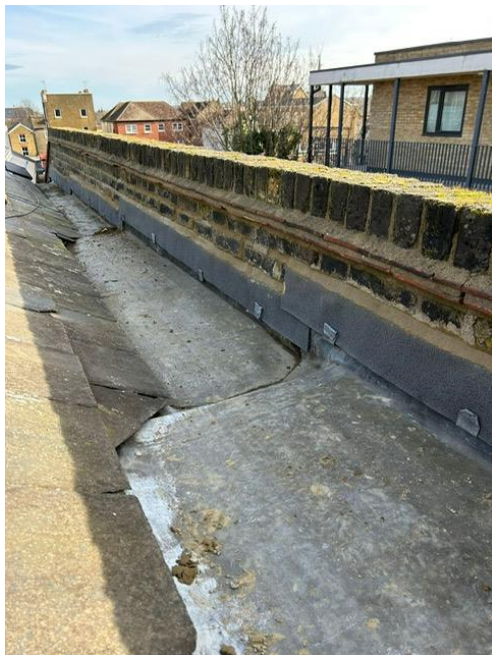
New / repair work to box gutters, roof junctions and valleys
