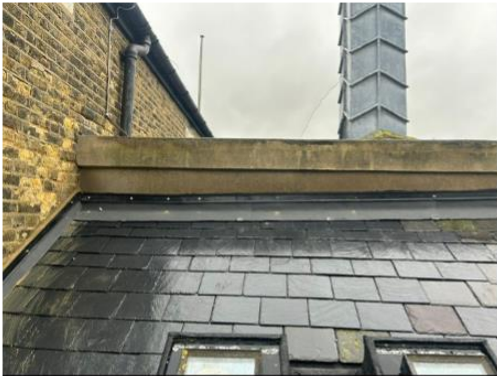
Slate repairs
