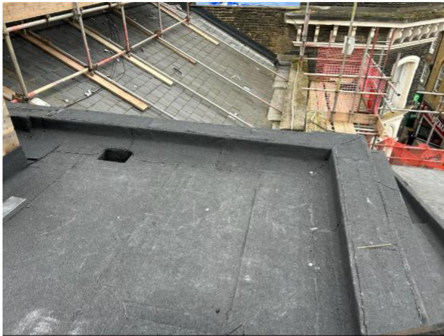
New flat roof
