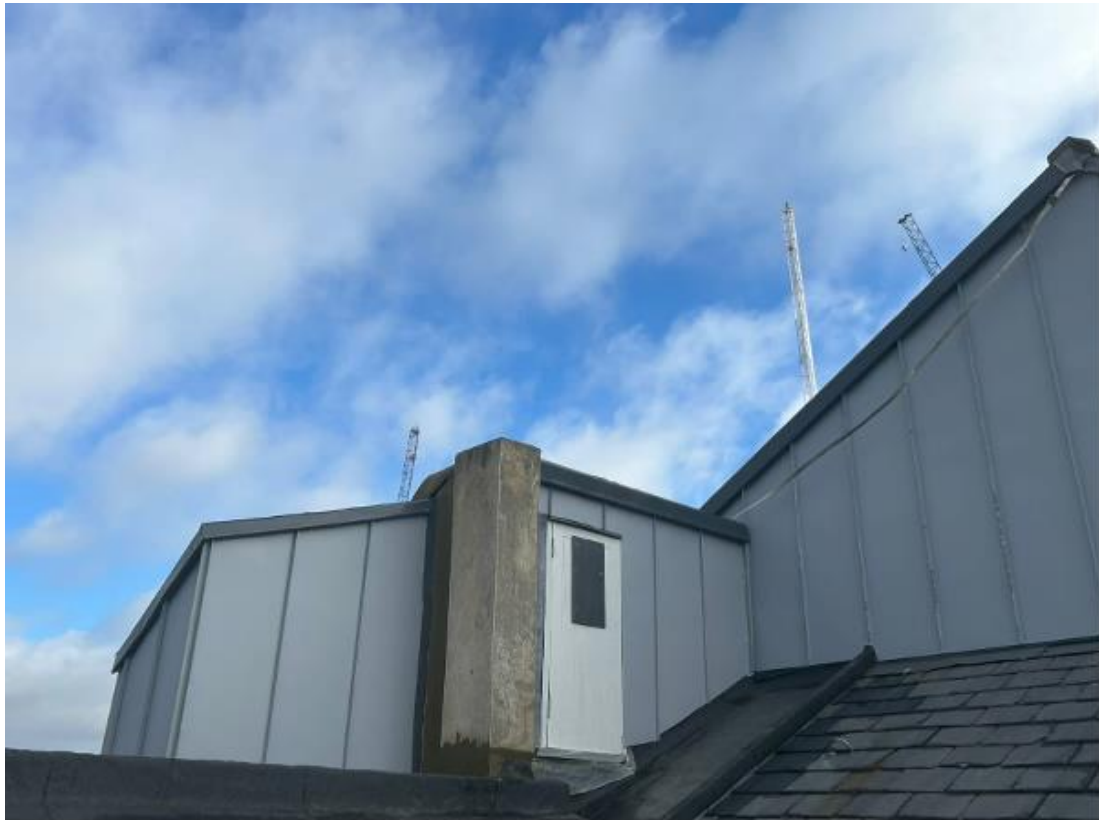
Standing seam zinc cladding (see Views 4 & 6 – pgs 8 & 9 for damaged roofs and gable end)
