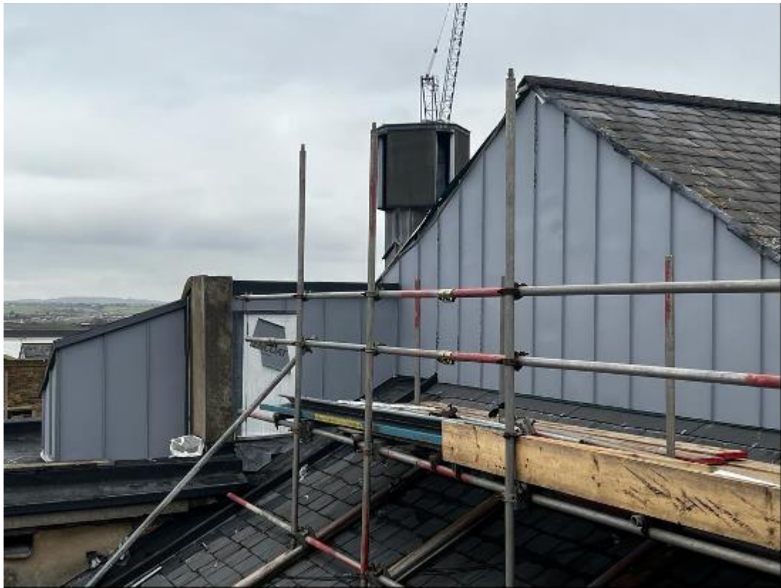
Standing seam zinc cladding (see Views 4 & 6 – pgs 8 & 9 for damaged roofs and gable end)
