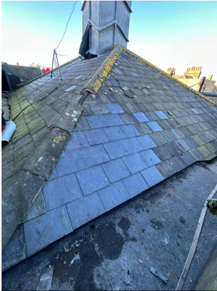
Slate repairs
