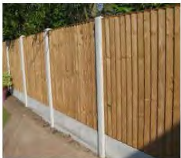
F2 : 2000MM HIGH TIMBER FENCE WITH 100X100MM CONCRETE POSTS & LOWER CONCRETE BOARD
