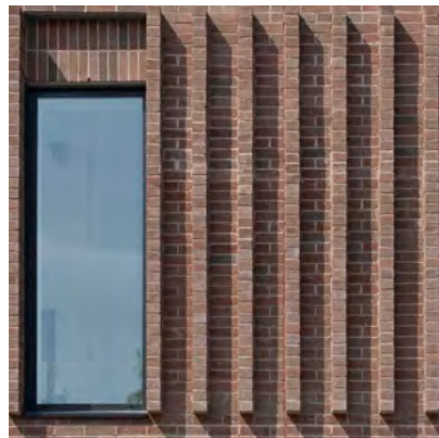
② Brick Detail - Protruding brick
