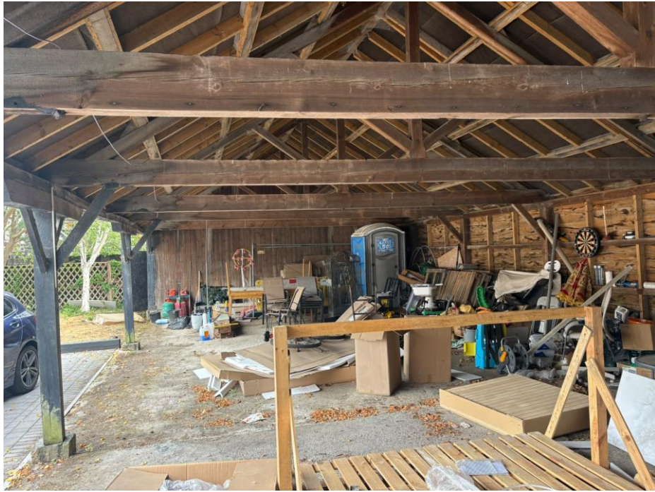
Photograph 3 – The internal aspect of the building.
