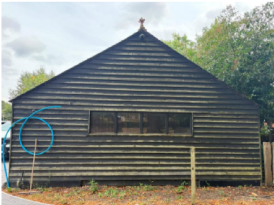
Photograph 2 – The west elevation of the building.
