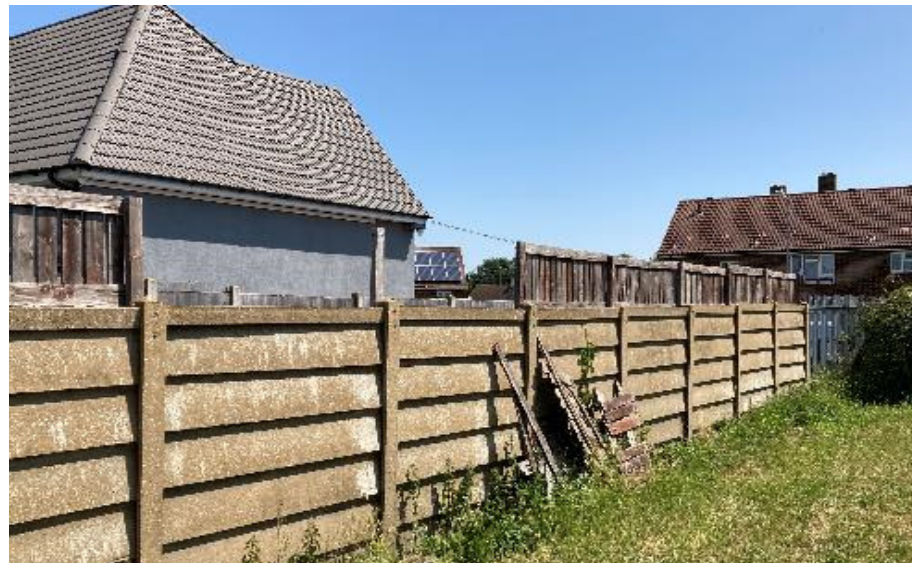
2. North boundary looking northeast
