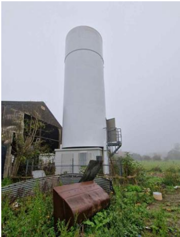
The imitation silo housing the telecommunications equipment is shown below:
