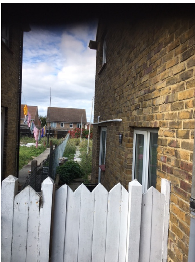
Fig iv: View of side access.
