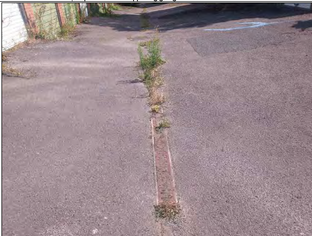
Photo 4: Site dipping down to a central drain run which ultimately dipped down to the east (facing east).
