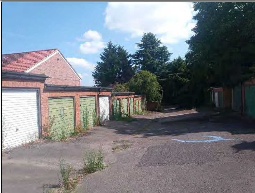
Photo 1: Two opposing rows of garages with hardstanding, facing east.
