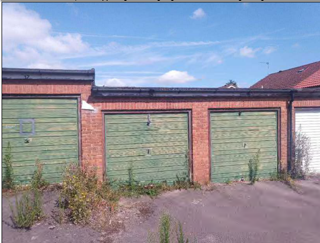
Photo 2: Garages of brick construction (facing north).
