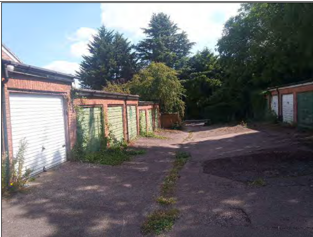
Photo 3: Dip down from opposing garages to centre of site.
