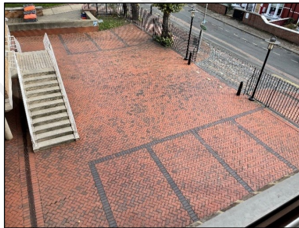
Figure 1: Existing Car park in front of main entrance
