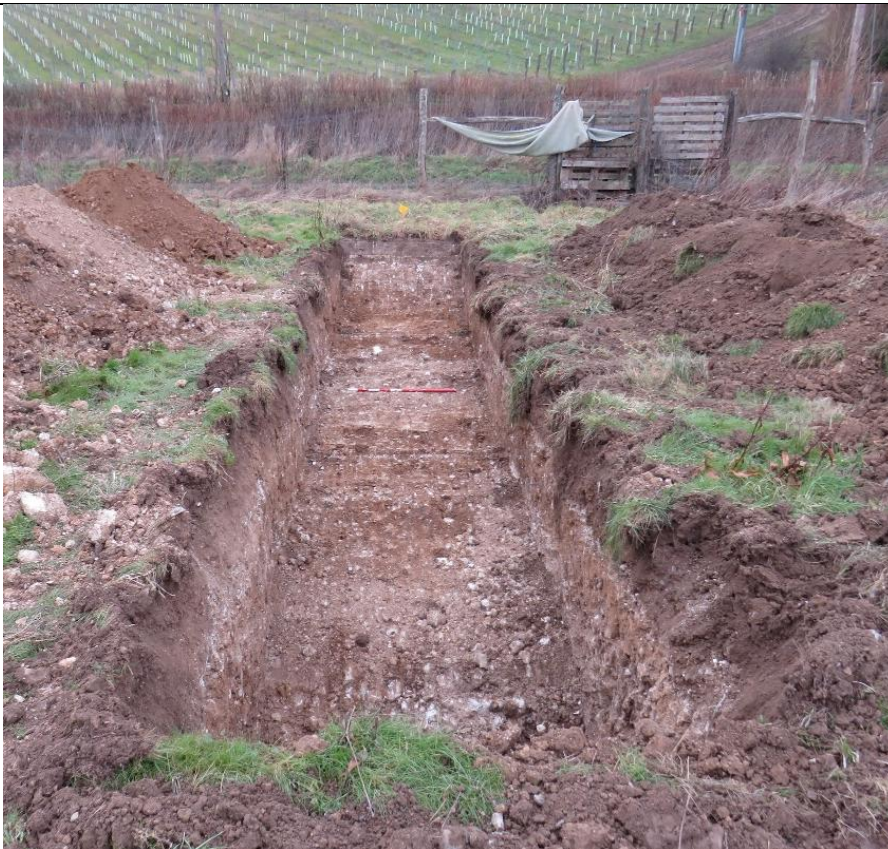
Plate 14. Trench 5, looking broadly north-west, downslope (scale 1m)
