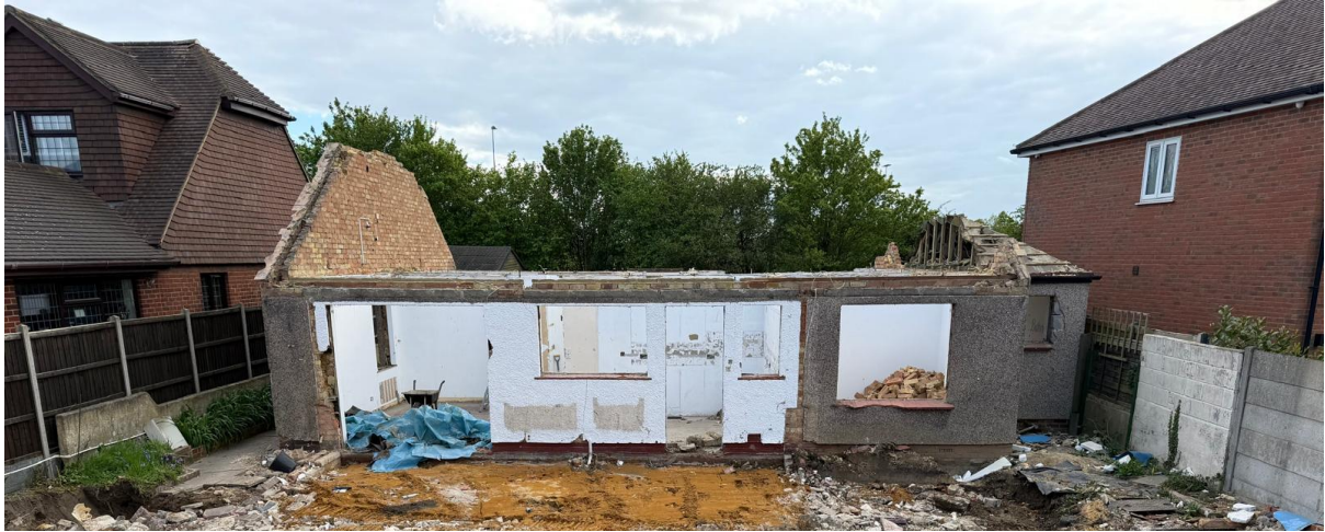
Figure 16. Existing dwelling following removal of the roof structure in accordance with the approved works
