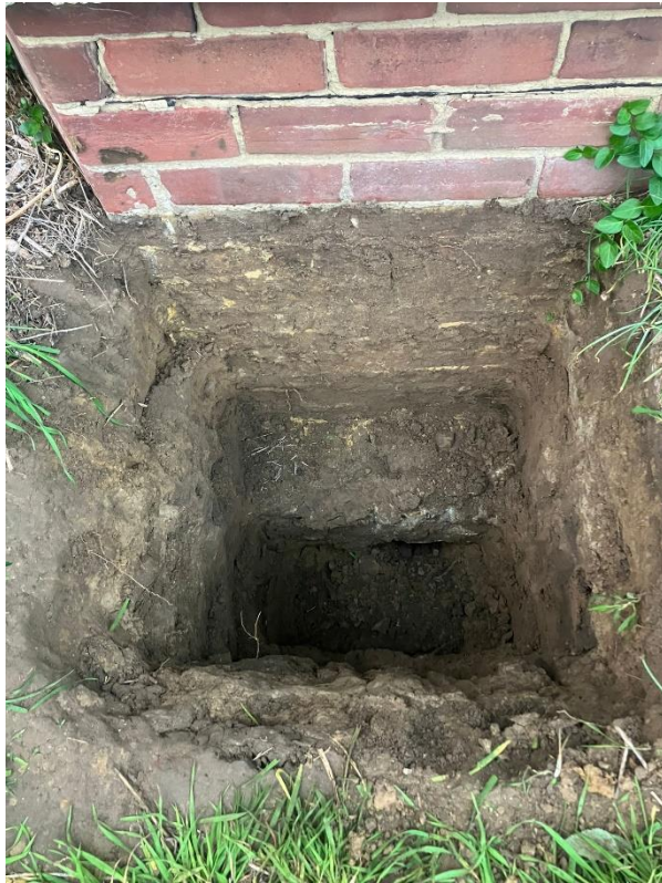
Figure 11. Trial excavation exposing the existing shallow strip foundation during the structural investigation
