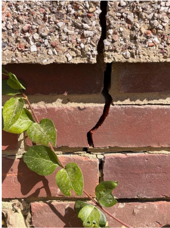
Figure 14. Significant structural cracking and movement to the external masonry wall identified during construction
