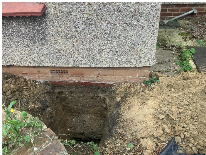
Figure 12. Trial excavation exposing the existing shallow strip foundation during the structural investigation
