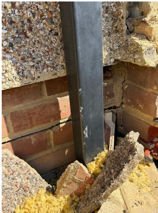
Figure 14. Significant structural cracking and movement to the external masonry wall identified during construction
