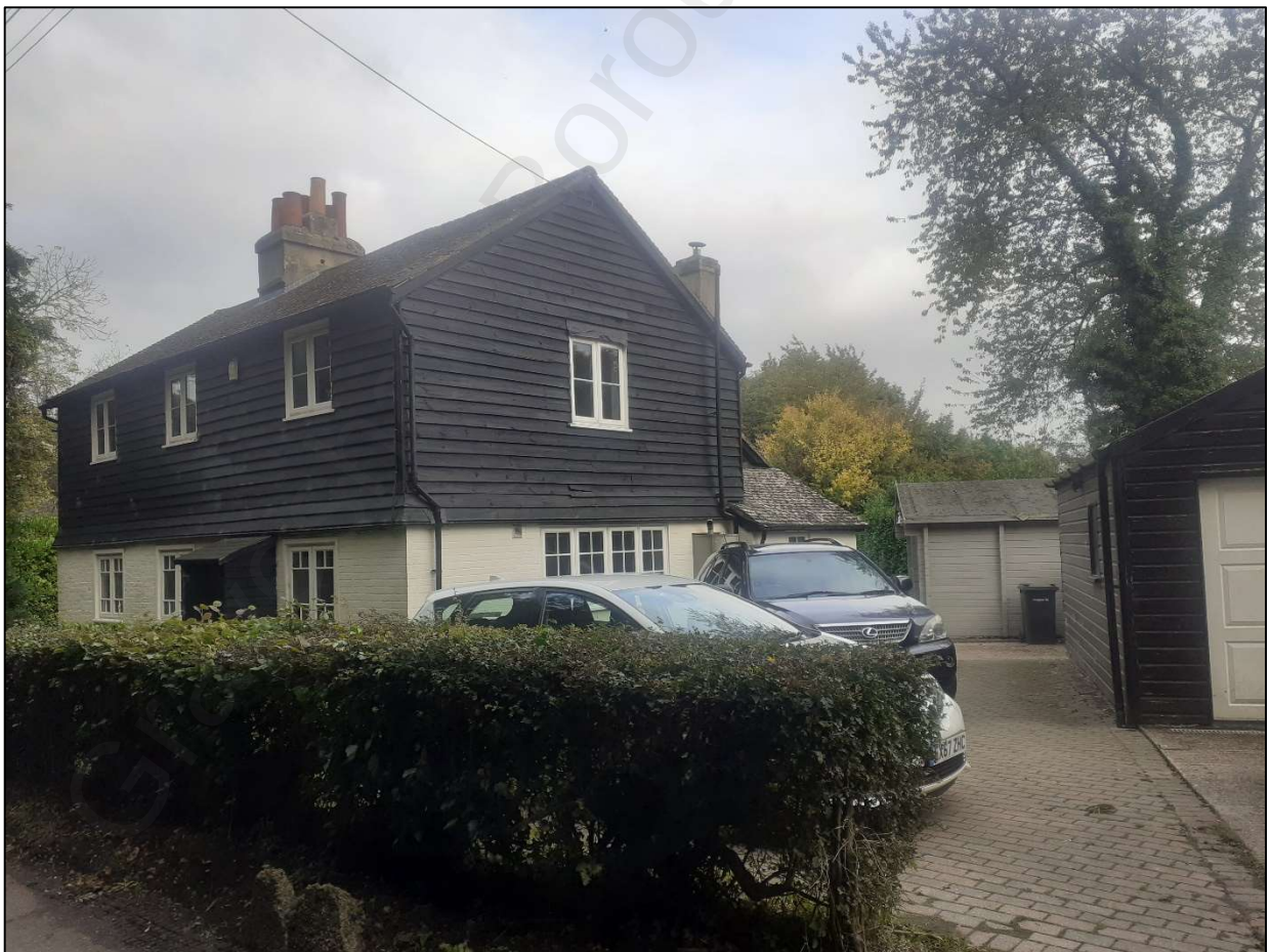
Figure 3: Front elevation of property and garage.
