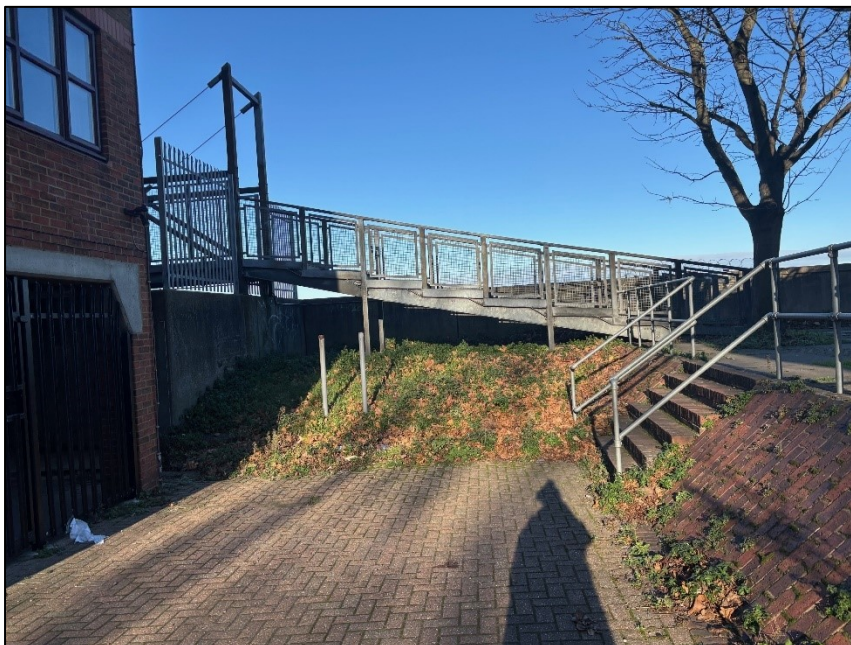
Figure 1: Existing grassed area at northern point of Elizabeth Gardens Access road.
