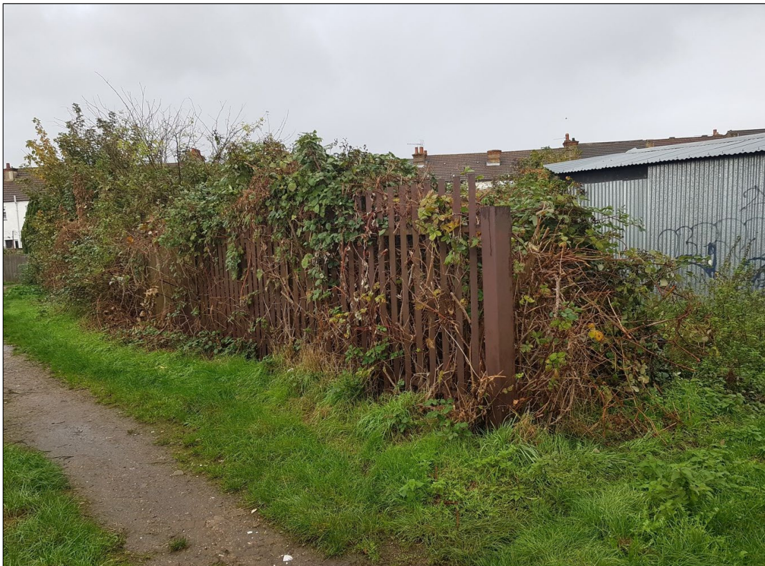
Figure 2. Southeast corner of site.
