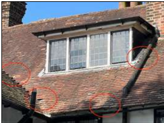
Photograph 11: Examples of PRFs on building B1.
