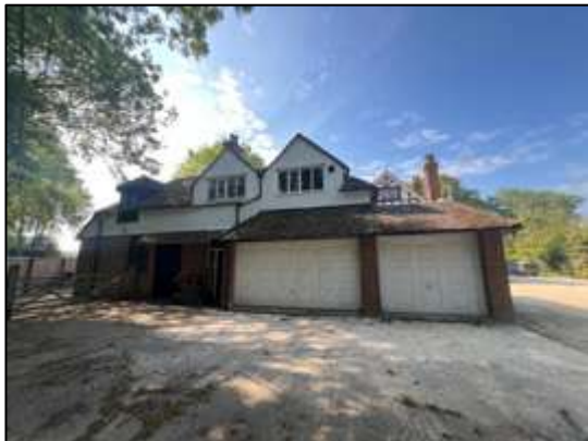
Photograph 3: B1a northern elevation.
