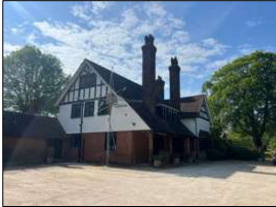
Photograph 1: Building B1 northern elevation..
