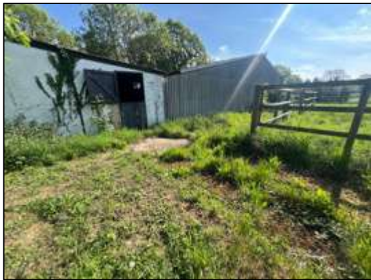
Photograph 27: Southern elevations of the stables and barn.
