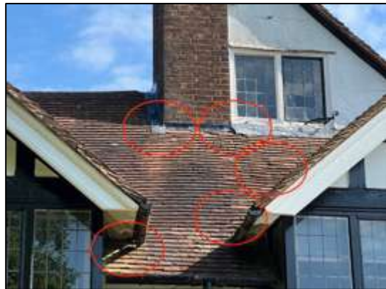
Photograph 12: Examples of PRFs on building B1.
