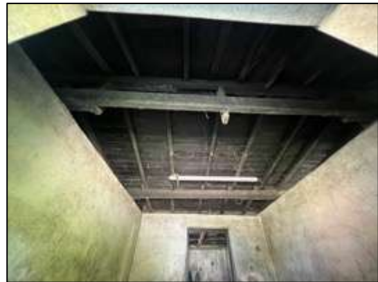
Photograph 18: Internal view of the stables.
