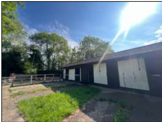
Photograph 17: Building B2, the stables.
