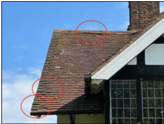
Photograph 9: Examples of PRFs on building B1.
