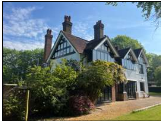
Photograph 10: Southern elevation of B1.
