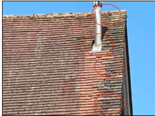
Photograph 8: Examples of PRFs on building B1.
