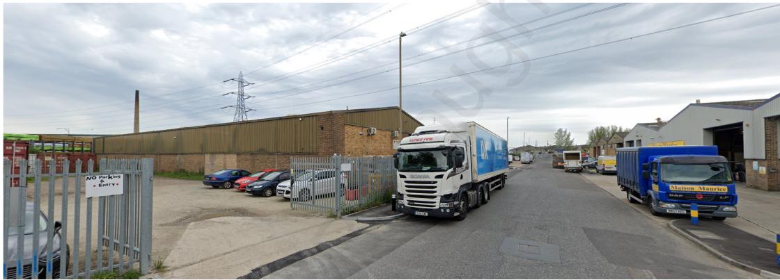
View of J1 building (right) from south west
