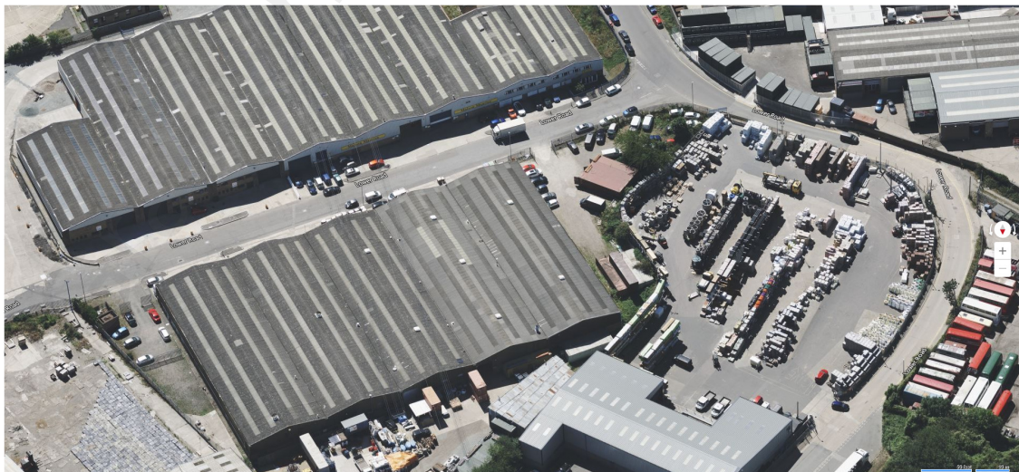
Aerial view of site from north, unit J1 on right
