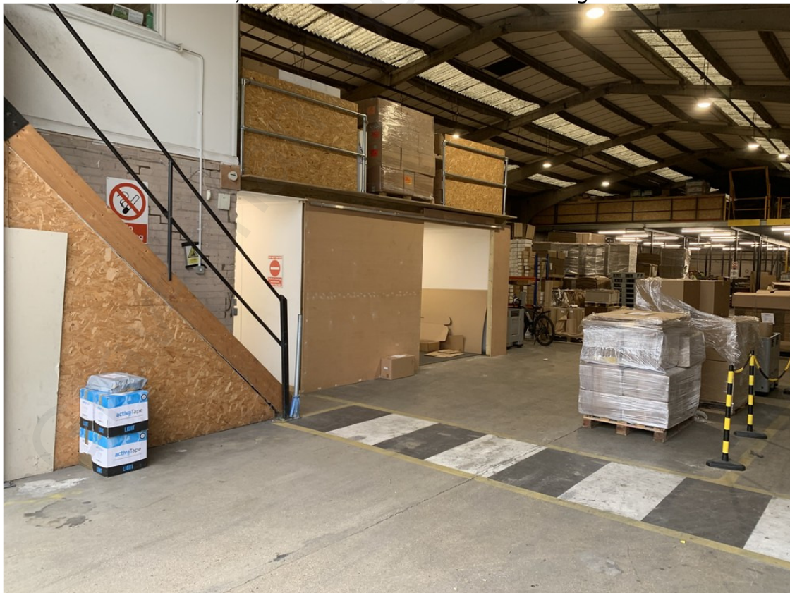
View of interior of main internal space.
