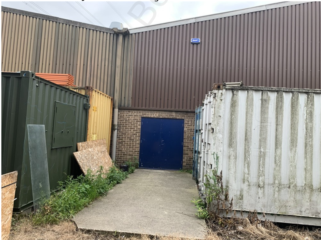
View of rear of J1 building
