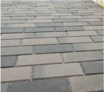
Permeable vehicular sett paving,
