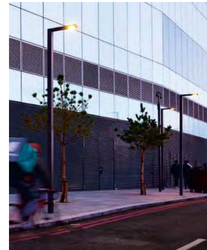
Street lighting columns
