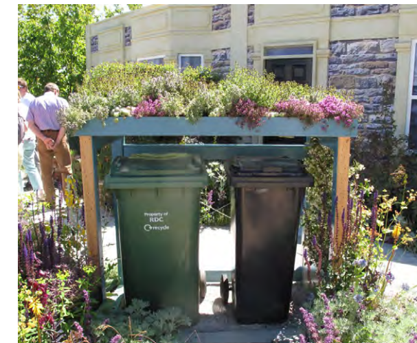
Green roof bins
