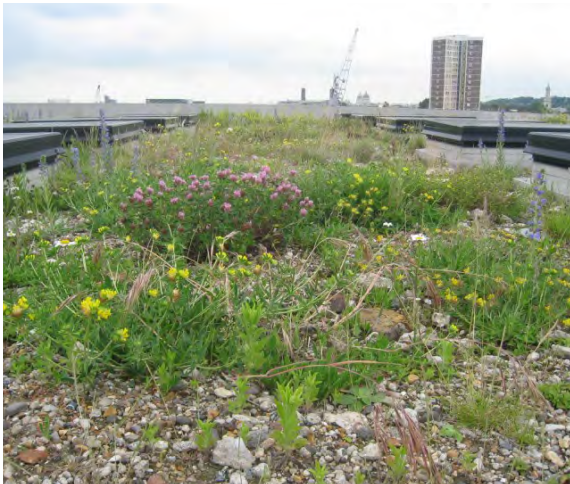
Planted green/brown roofs
