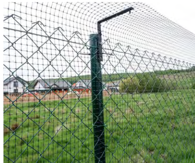
Provision of cat-proof fencing at the boundary adjacent to the SSSI
