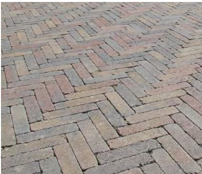
Clay block paving
