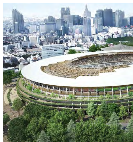
Japan National Stadium - Kengo Kuma
