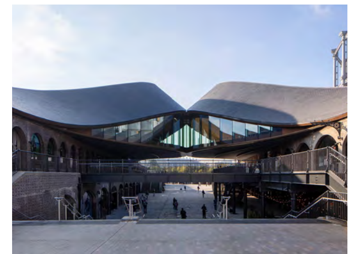
Coal Drops Yard - Heatherwick Studio
