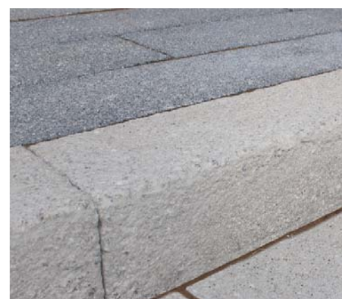
Pre-cast grey concrete kerb
