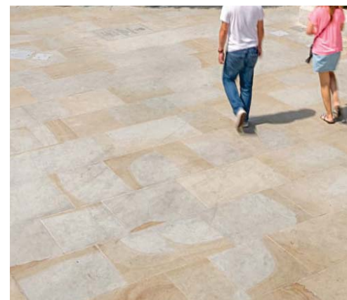
Yorkstone paving flags, stretcher bond
