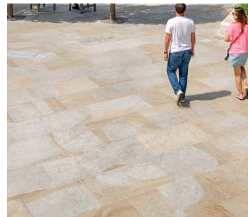
Yorkstone paving flags, stretcher bond
