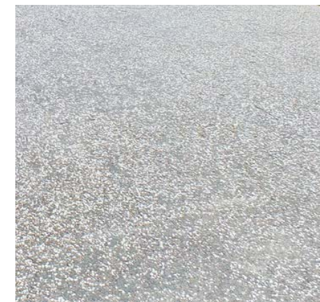
In situ exposed grey aggregate poured concrete
