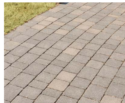
Tegula permeable paving setts, various sizes, stretcher bond
