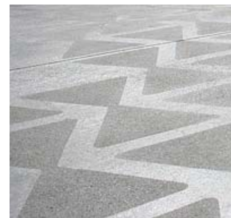
Sand blasted surface
