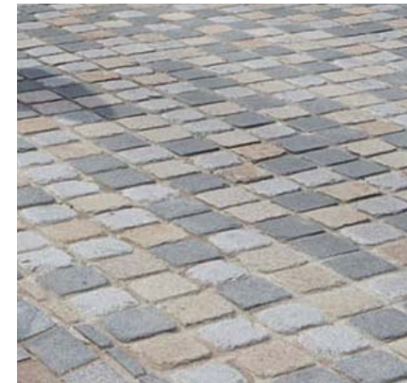
Tumbled vehicular sett paving, stack bond
