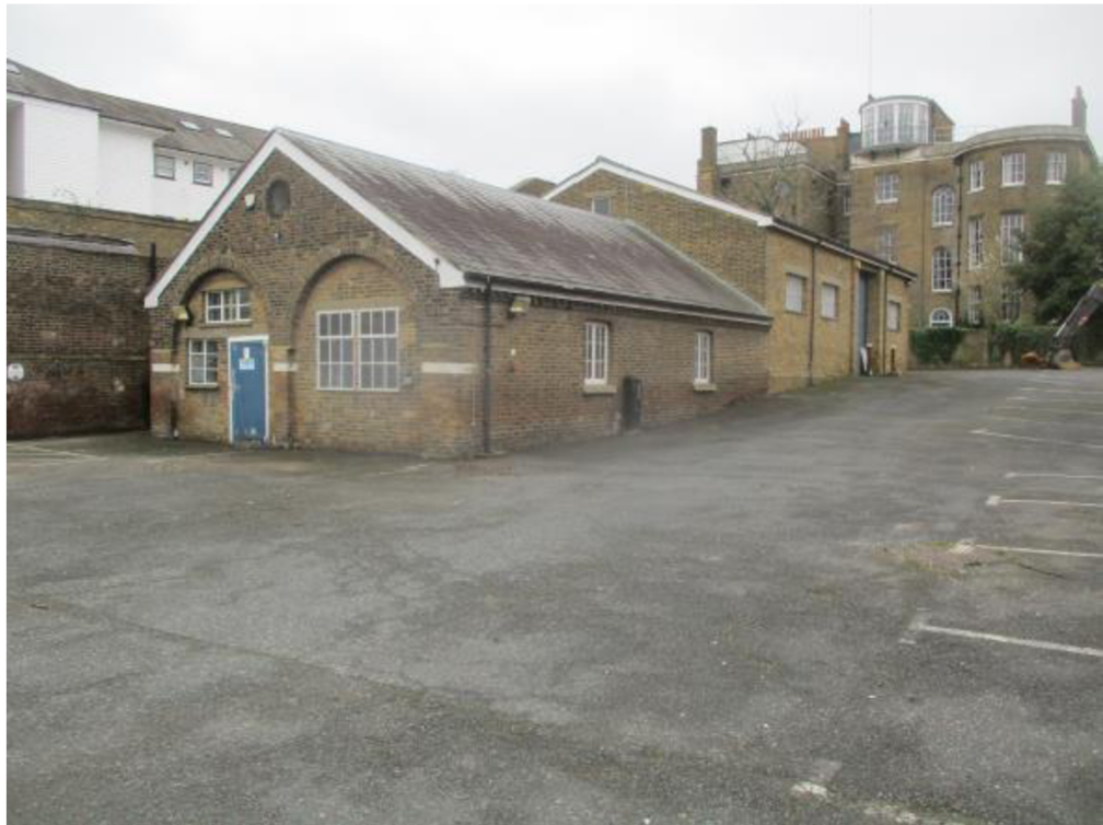
Plate 3. The Custom House boathouse with blocked arched entrances and a later workshop to the rear and with Custom House in the background
