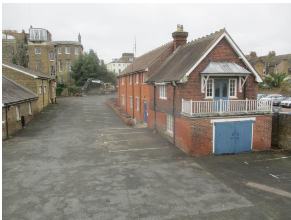
Plate 5. The red-brick ancillary buildings to the west (looking south)
