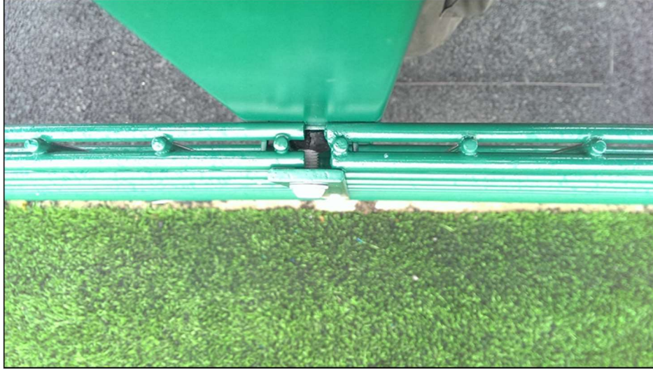
Figure 10: Image Showing Neoprene Isolators
