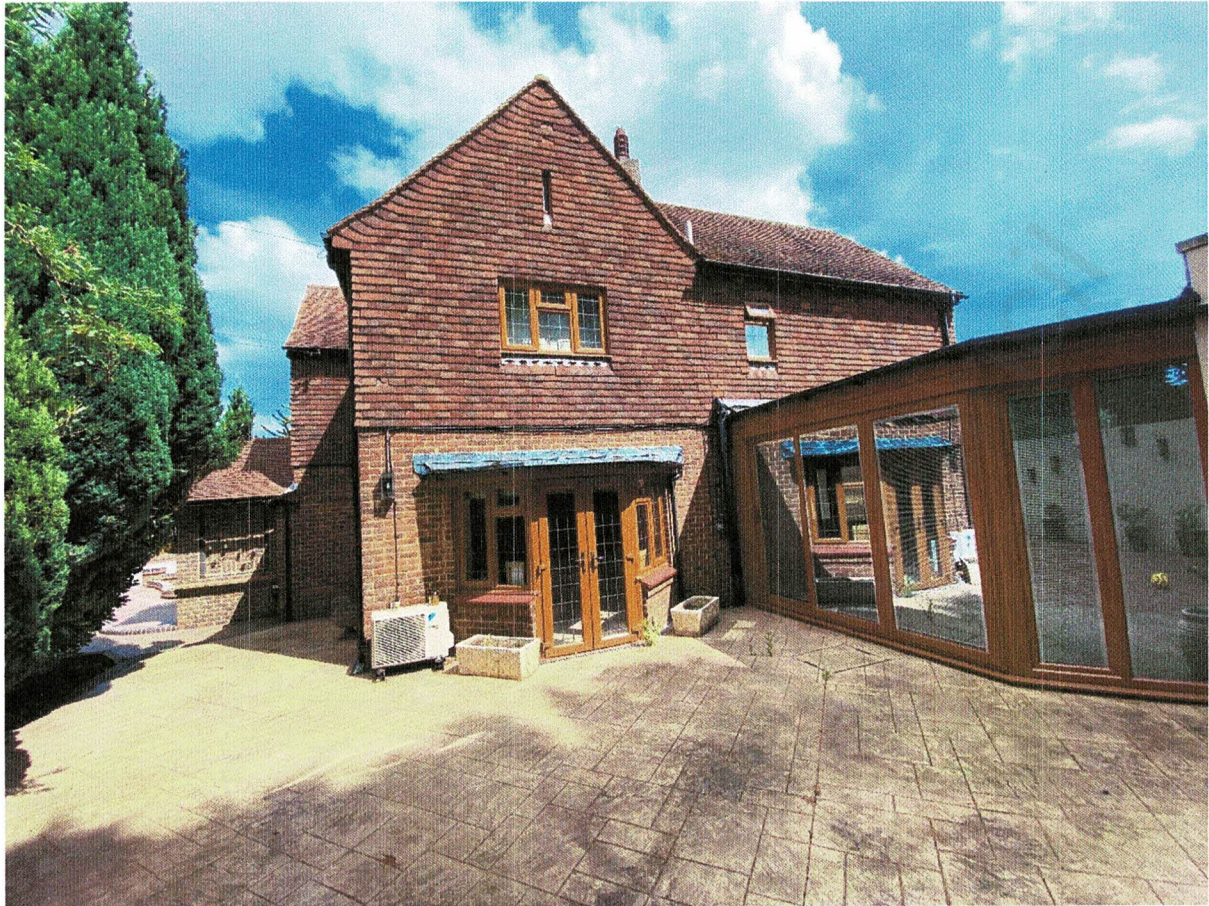
Southern elevation which shows the porch extension on the left side of the photograph, the side extension on the right side.
