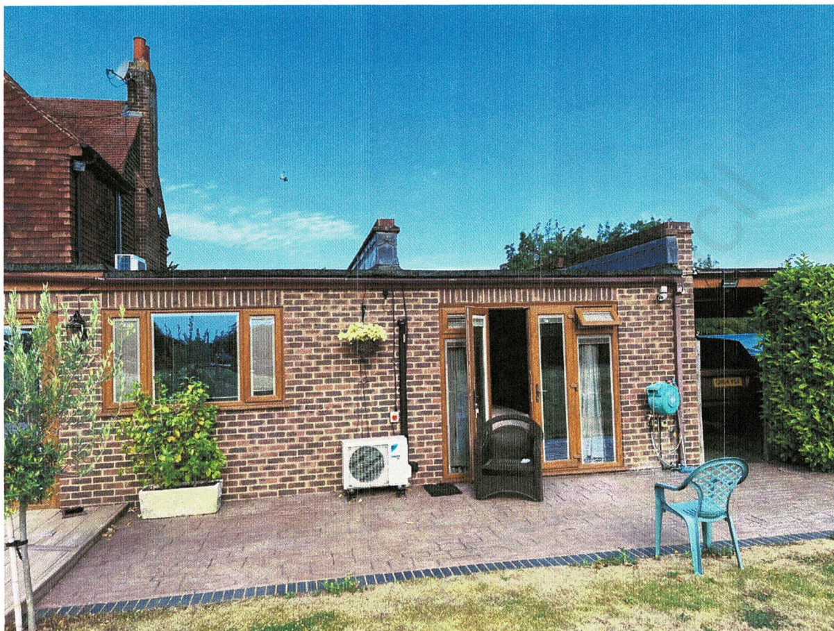
Rear elevation formerly the garages and now part an annex and part kitchen
