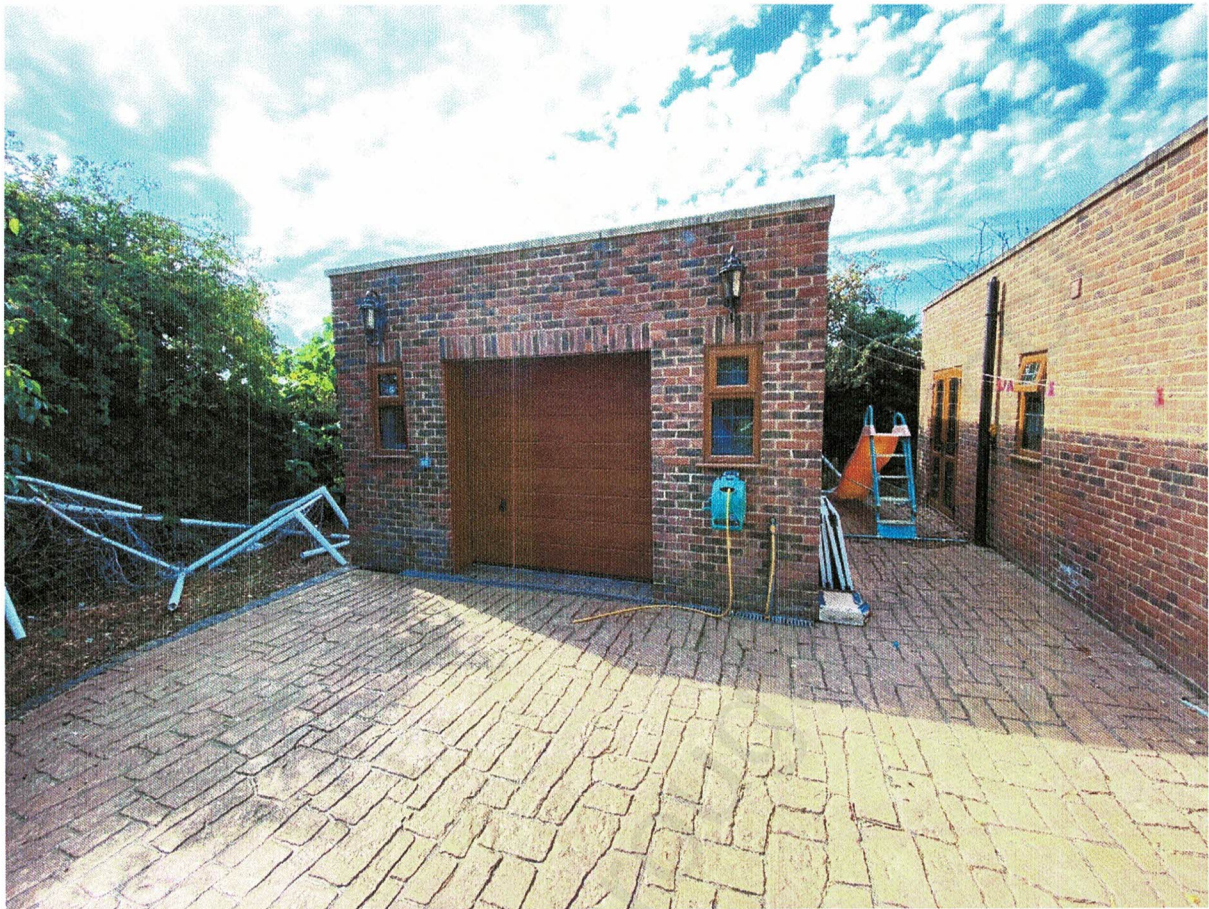
Single storey store to the rear of the pool room.
