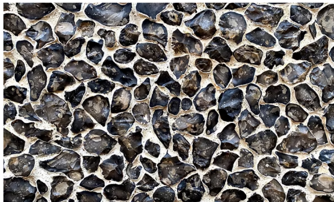
fig - 001 napped flint wall to tie into existing house
