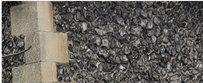
fig – 002 flint wall with stone quoins
