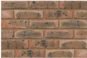
Ibstock Brick - Chailey Red Stock with matching soldier course bricks over at 215mm high
