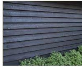
Black stained feather edge timber weather boarding
