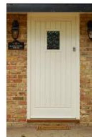
Doors - white painted timber frames and panels with single viewing panel centered.
