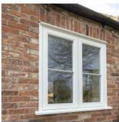
Windows - white painted timber double glazed with white timber cills and single timber glazing bar
