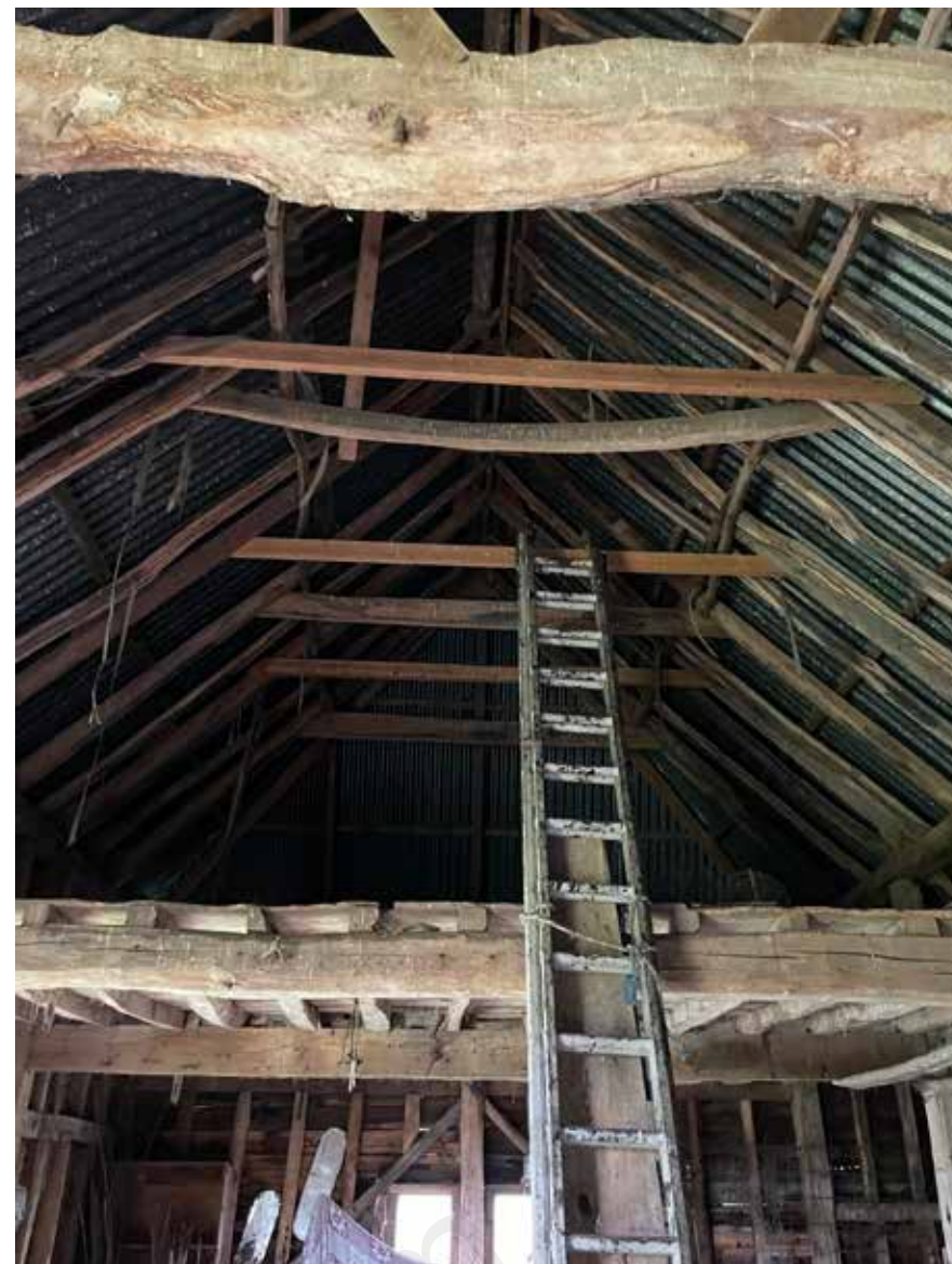
Current - Mezzanine level
