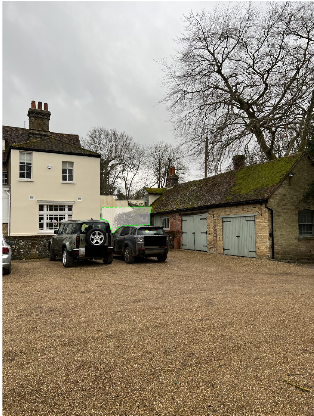
Position of new north-facing wall (highlighted) of the proposed link extension, as seen from this private vantage point.
