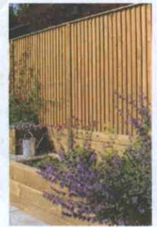
Timber Fencing between units
