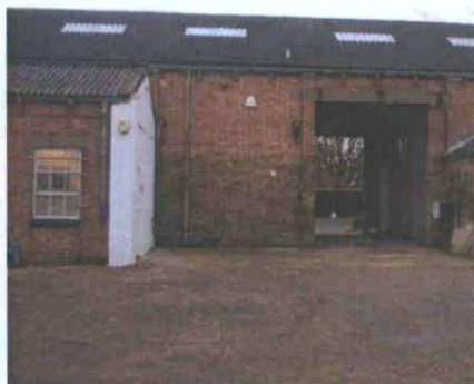
Image of existing industrial building
