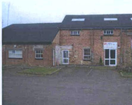
Image of existing industrial building
